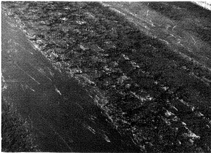
Figure 5. Tearing of Gussasphalt by paver screed because of low mix temperature.
