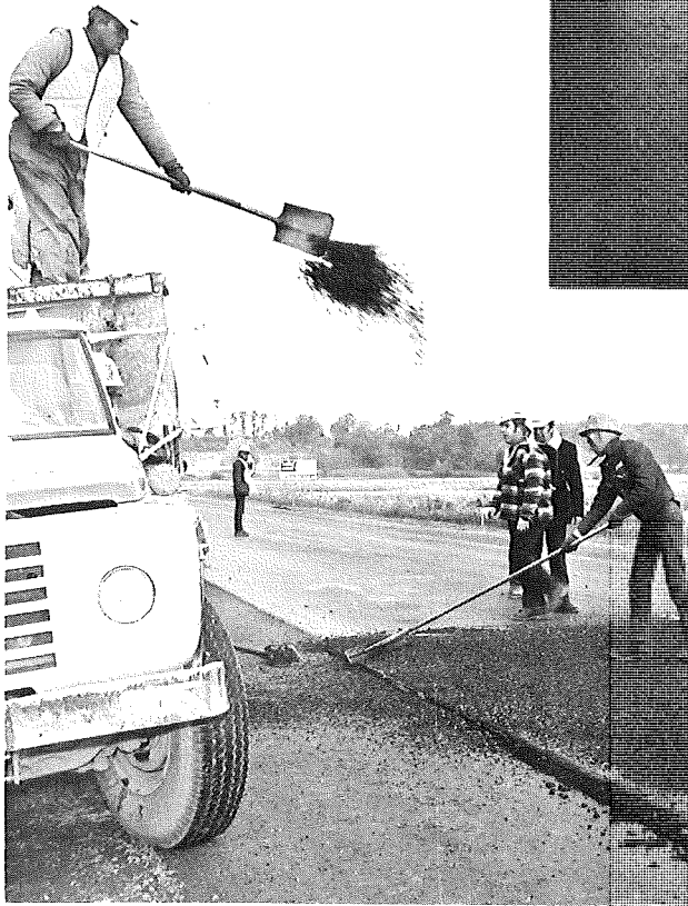
Figure 8. Spreading cover stone on Gussasphalt.
