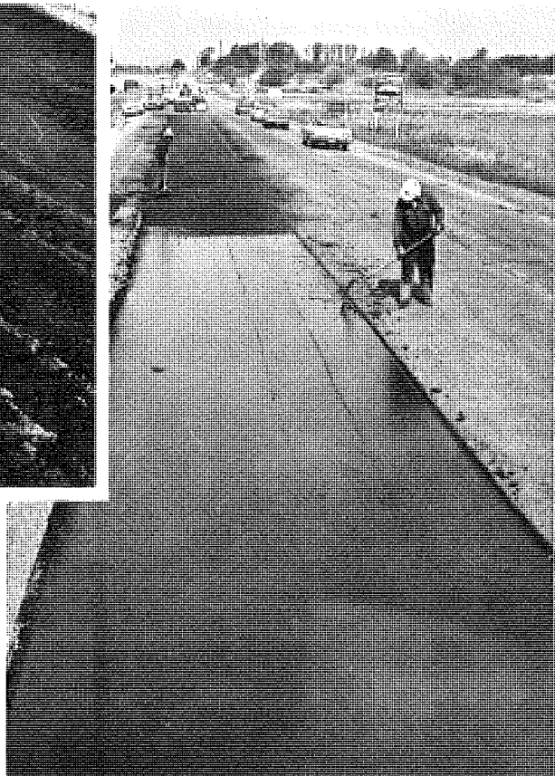
Figure 5. Tearing of Gussasphalt by paver screed because of low mix temperature.
