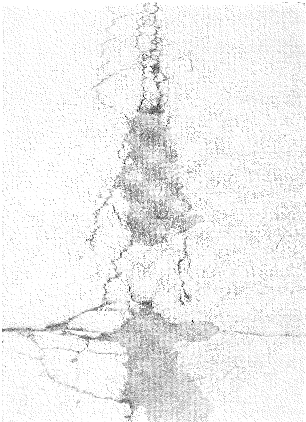
◀ Figure A3. High-Severity Longitudinal Joint Reflection Cracking.
