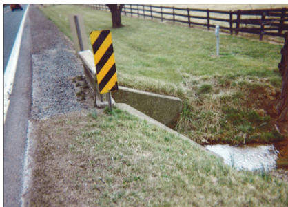
Rigid headwall delineated with Type 3 Object Marker.
