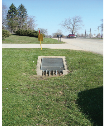
This grated inlet can be used to prevent water ponding at access points.
