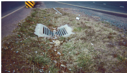
V-shaped grate in median.
