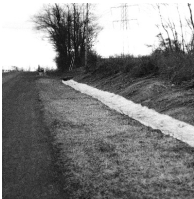
Erosion control measures such as fiber mats shown may be necessary to prevent ditch erosion.
