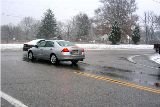
Water ponding in wheel ruts.
