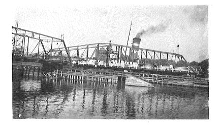
Swing Bridges are pivoted in the middle and can be turned parallel with the stream. Three swing bridges on I-94BL are located at St. Joseph-Benton Harbor and South Haven. Another is on M-64 at Ontonagon and a fifth at St. Clair on M-29.
