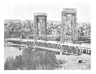
THE HOUGHTON-HANCOCK BRIDGE is a double-deck, lift span with a four-lane highway on the upper level and a railroad track on the lower level. It can be raised like an elevator to a height of 100 feet above the water. When neither trains nor large boats are expected, the railroad level can be raised to the auto level permitting auto traffic to cross on the railroad deck while small boats pass underneath.
