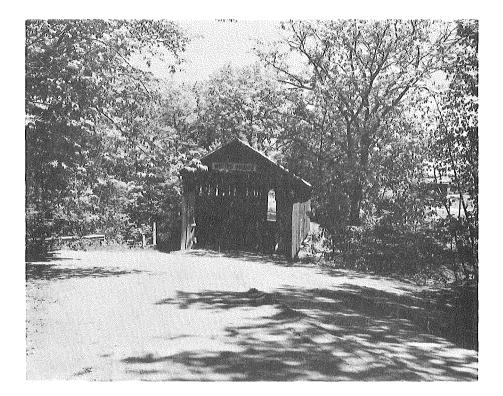
WHITE'S BRIDGE located in Ionia County just east of the Kent County line was built in 1867 by Jared N. Brazee and J. N. Walker. It is 14 feet wide and 116 feet long, cost \$1,700. It is of the through-truss type with a gable roof. The hand-hewn trusses are sheeted over with rough pine boards. Wooden pegs and handcut square iron nails were used to secure the various parts of the bridge. White's Bridge has been in constant use since 1867, proof that it was well constructed.
