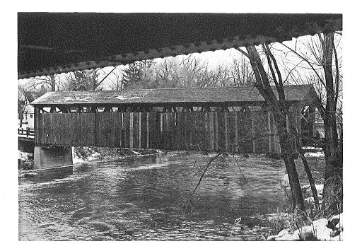
The Ada Bridge was built by Will Holmes, and is 125 feet long and 14 feet wide. It was opened July 7, 1867, and was nearly wiped out in the floods of 1904 and 1905. Local old-timers remember how farmers saved the bridge by driving onto it with wagons loaded with stones. When it continued to sway in the current, boards on the sides were removed and the river was allowed to flow through. As an added measure, a heavy cable was tied to the bridge and snubbed to a nearby elm.
