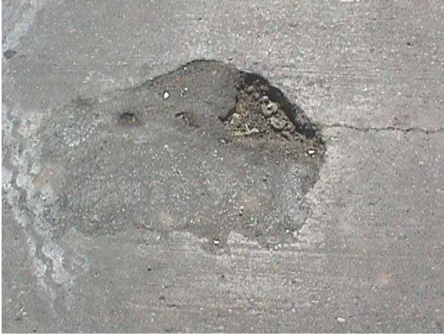
Figure 3-6. Pothole on the Way of Major Crack.
