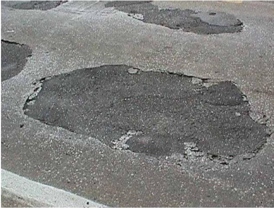
Figure 3-8. Potholes on the Way of Wheels.
