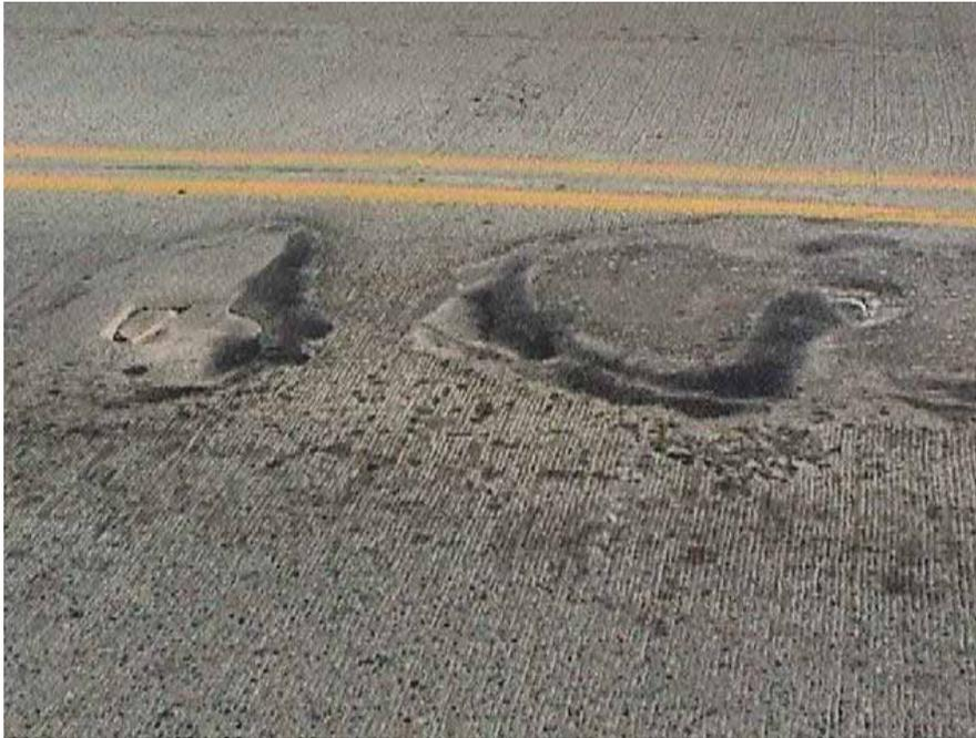
Figure 3-4. Potholes in Latex Overlay.
