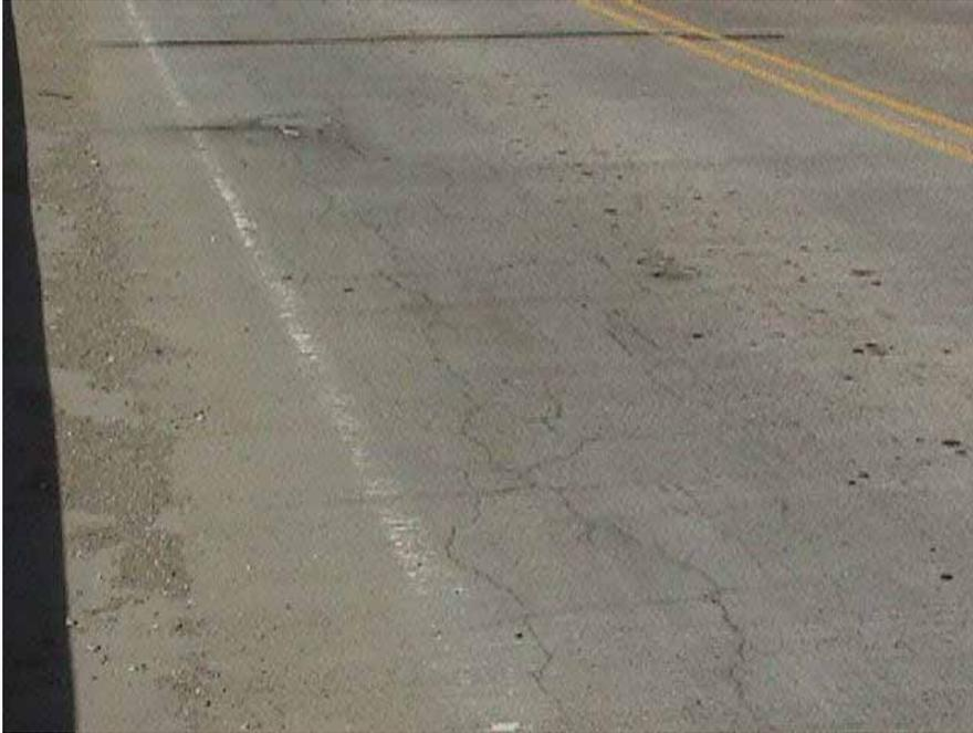
Figure 3-2. Longitudinal Cracks.
