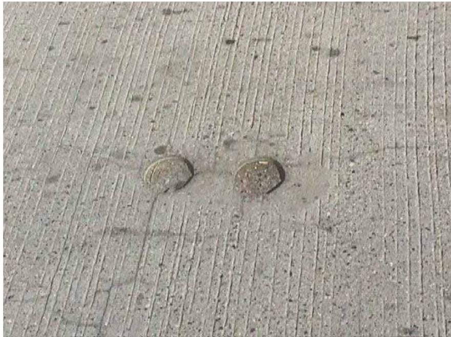
Figure 3-3. Cracks in Latex Overlay; Core Samples.
