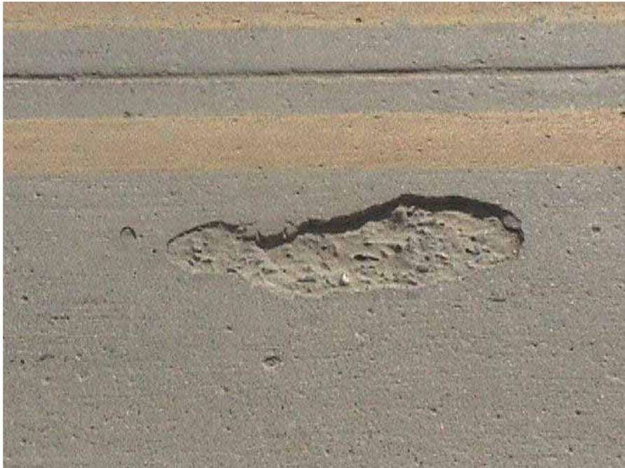
Figure 3-7. Pothole in Latex Overlay.
