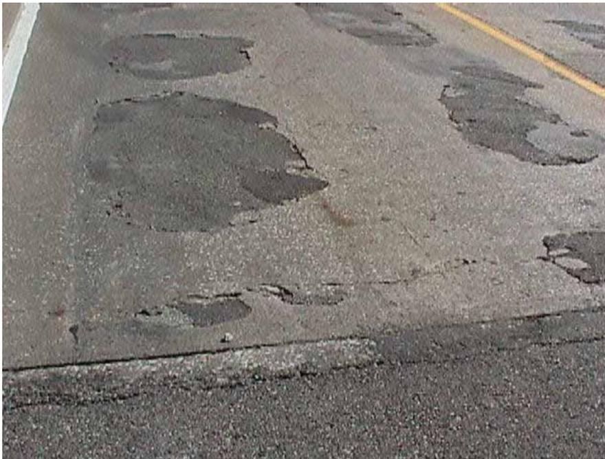
Figure 3-9. Holes on the Way of Wheels; Cracks Close to Joint.
