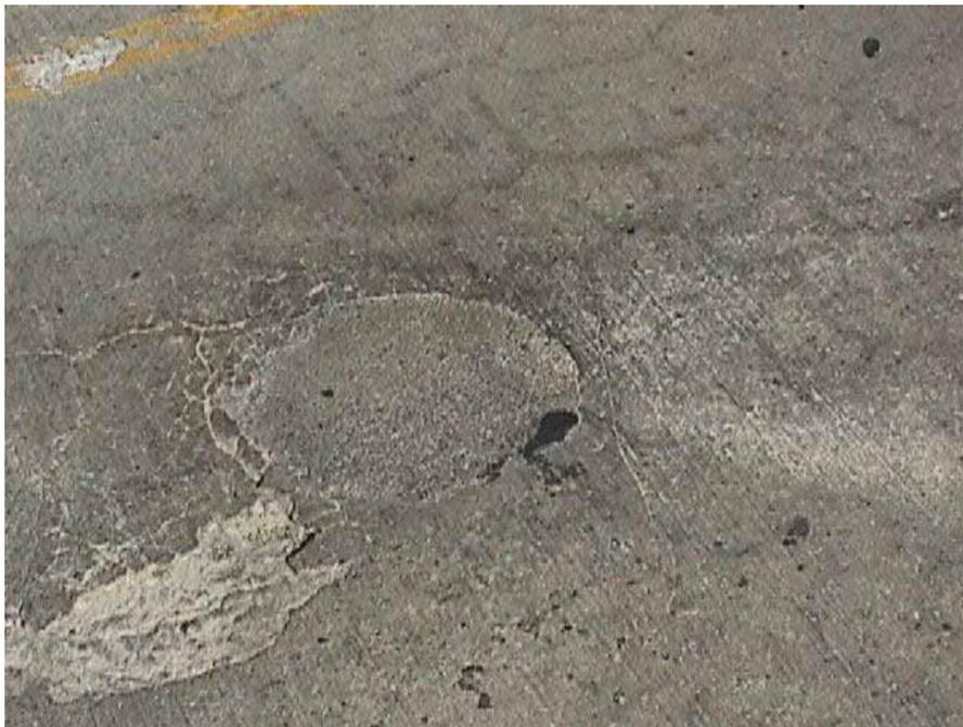
Figure 3-5. Pothole with Map Cracks.
