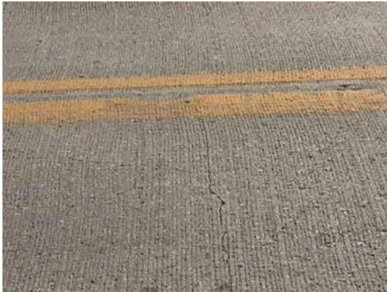
Figure 3-1. Transverse Shrinkage Cracks.
