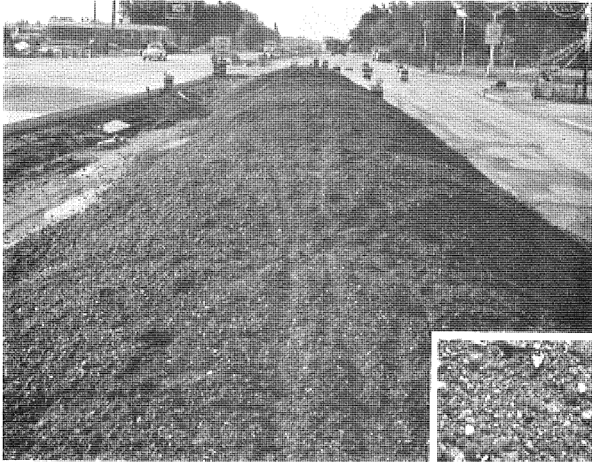
▲ Stockpiled cold-mixed emulsion black base material.
