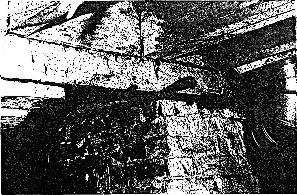
Figure 1. Wooden beam supported by chimney. Note the wooden shims installed to fill gap of missing mortar.
