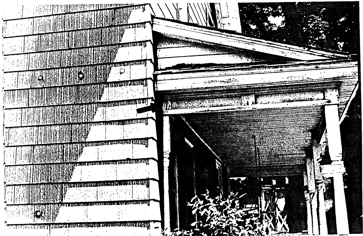
Figure 5. Porch pulling away from house approximately 1-1/2 inches due to settlement of its foundation.
