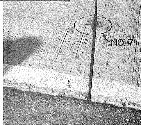
Figure 4. Cores taken from the non-draining bituminous base sections of the Clare Test Rd. The pavement was four years old when sampled. Core No. 1 is from an unfaulted westbound section, the other two are from the faulted eastbound section. All show the same heavy surface deterioration, evidently due to freeze-thaw action while standing in water. The faulted joint shown is the one from which Core No. 7 was taken. Note also the open shoulder-pavement joint.
