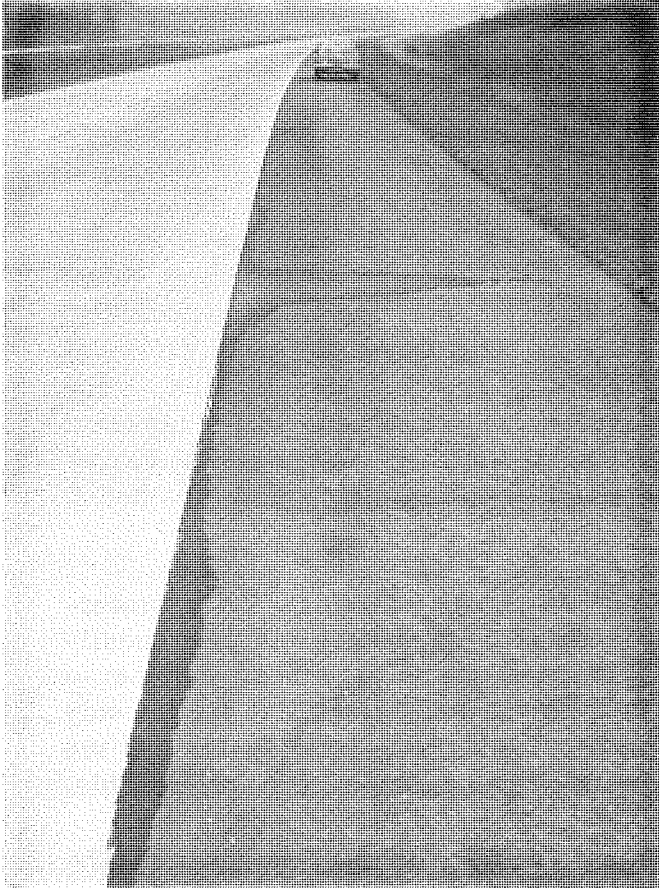
Figure 1. Eastbound superelevated bituminous base section. After rainstorm, water rises through shoulder-pavement joint and drains across surface of shoulder.
