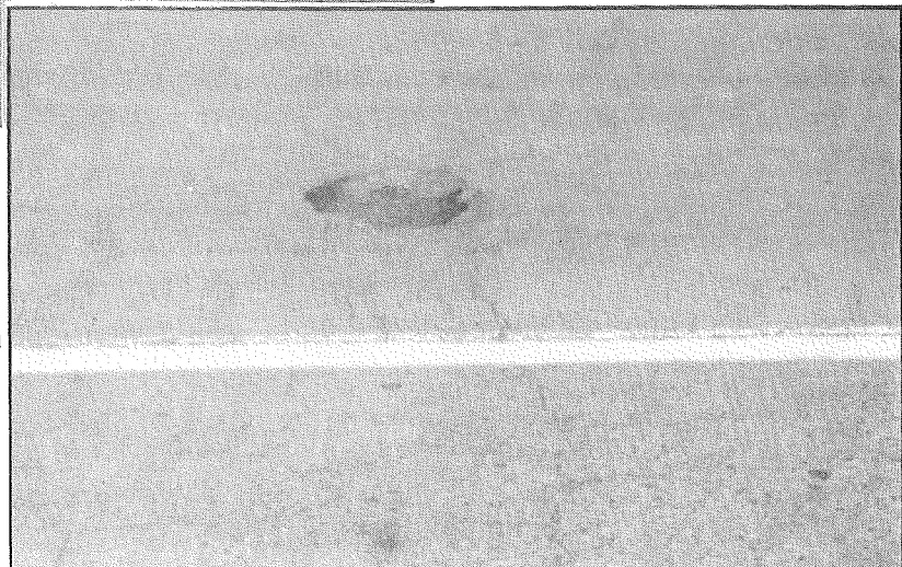
Figure 4. Surface repair in overlay on S10 eastbound.
