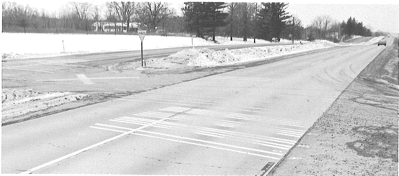
Figure 2. Terminal condition of test lines after 6-1/2 months of service.
