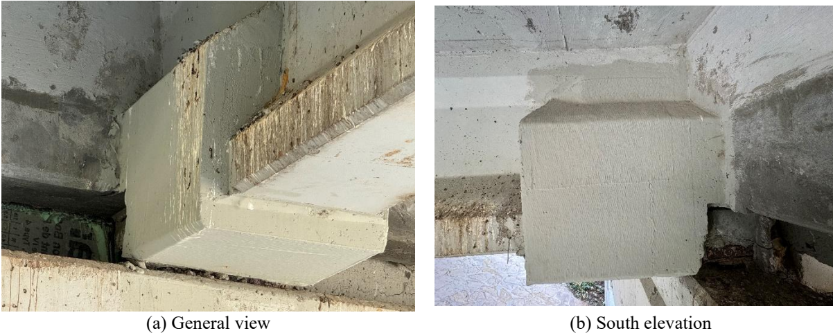
Figure D-67. The overcast with CFRP wrapping at beam 4s in span 1w at pier 1w as of 10/04/2024.
