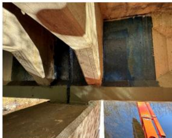
(c) Beam end with partial-height repair, FRP, and CSC
