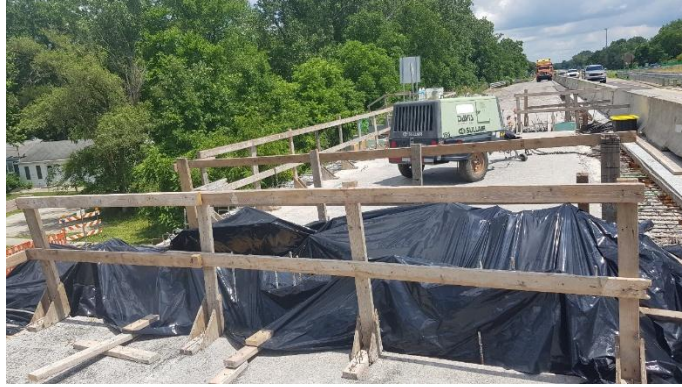
Figure F-18. Covering the concrete after placement.
