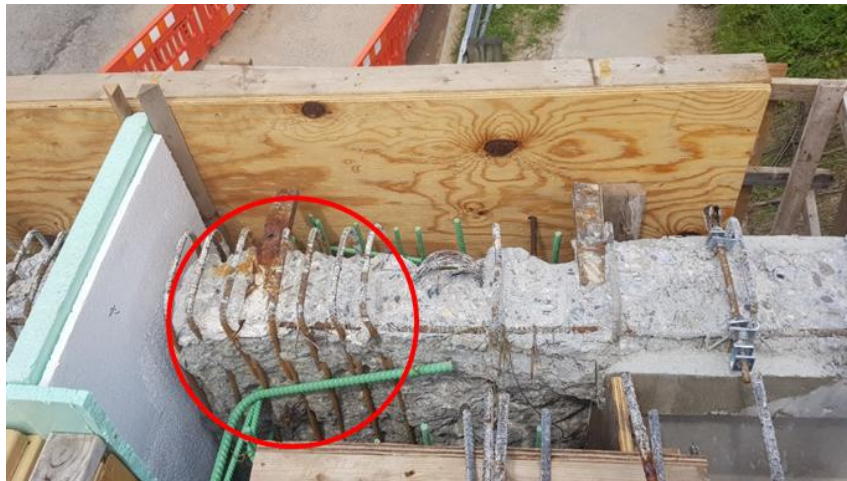
Figure F-21. Corrosion was observed on the existing reinforcement before pouring concrete.
