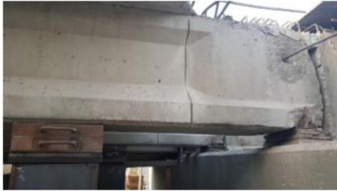
(b) Saw cut showing the section to be chipped out and cleaned
