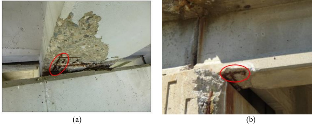
Figure 4-24. Section loss at the beam soffit with exposed strands and stirrups.
