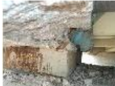
(b) Beam 8w in span 2s at pier 1s - spall with 13% LOB
