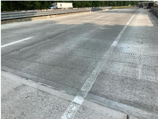
(a) General view of the bridge
