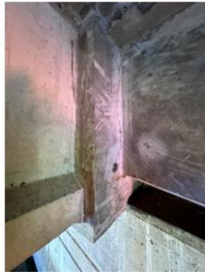
(b) Unreinforced concrete full-depth overcast
