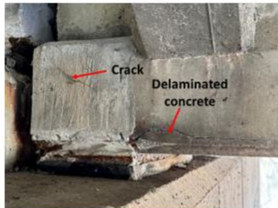
(f) An example of a repair performed without removing all delaminated concrete
