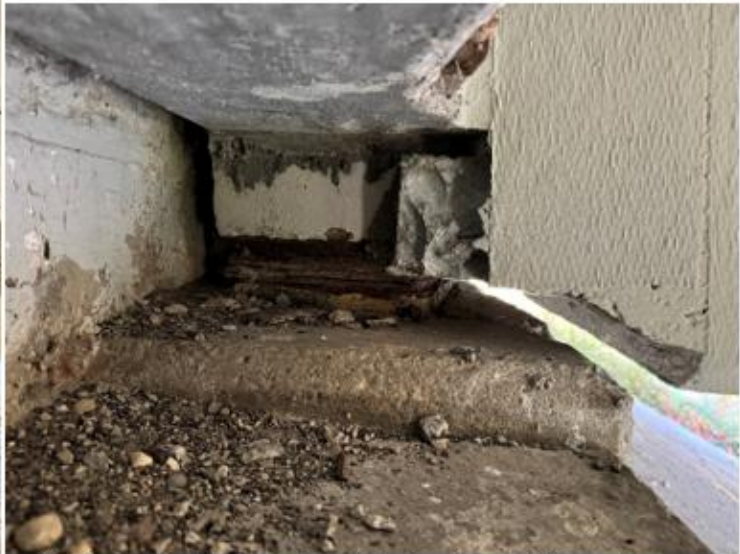
(b) Close-up of beam end showing bearing and the section over bearing without overcast
