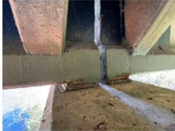
(b) Corroded sole plate and bearing plate promoting deterioration
