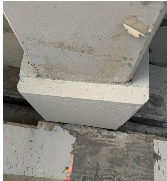
(b) Bottom flange soffit
