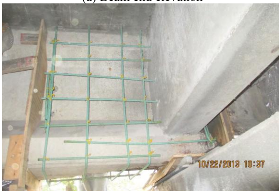
(c) Interior face of the fascia beam with end diaphragm
