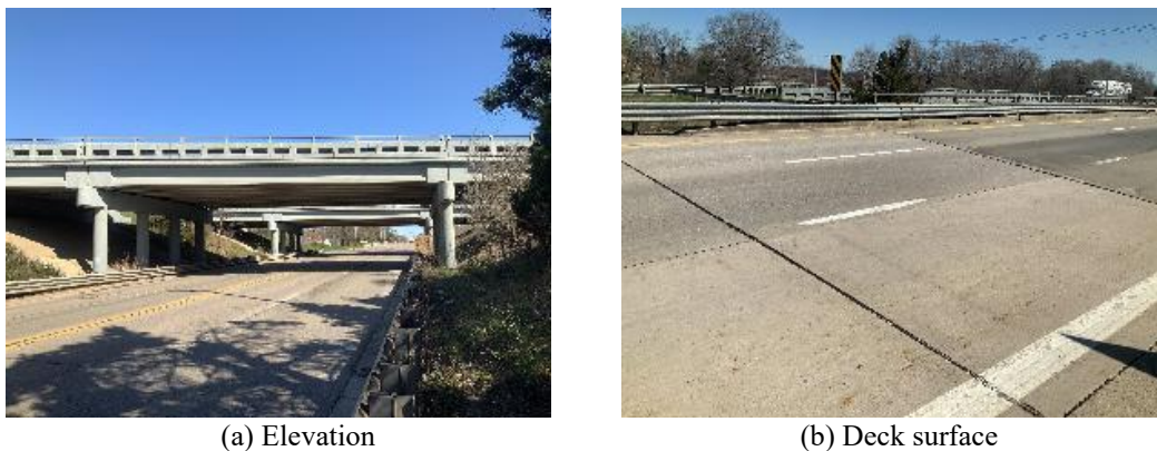
Figure D-3. I-69 Bridge over Linden Road.
