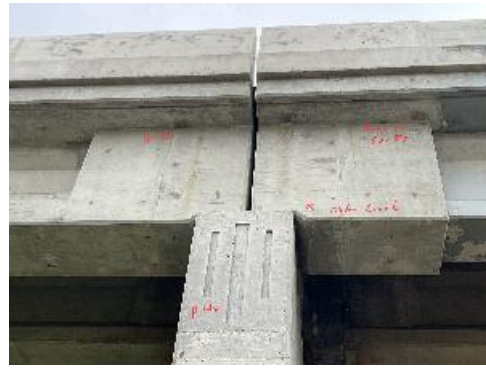
(b) Beam 6w in span 5s at pier 4s – tight crack
