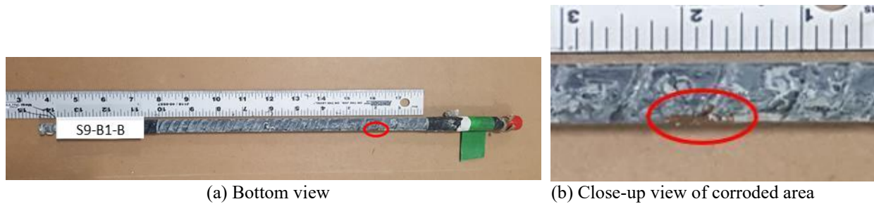
Figure 5-17. Condition of Rebar-1 from S9 specimen.
