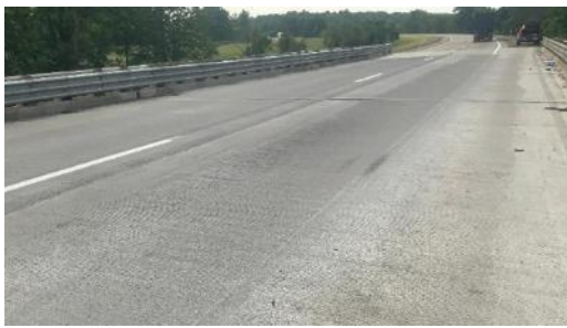
(a) General view of the bridge
