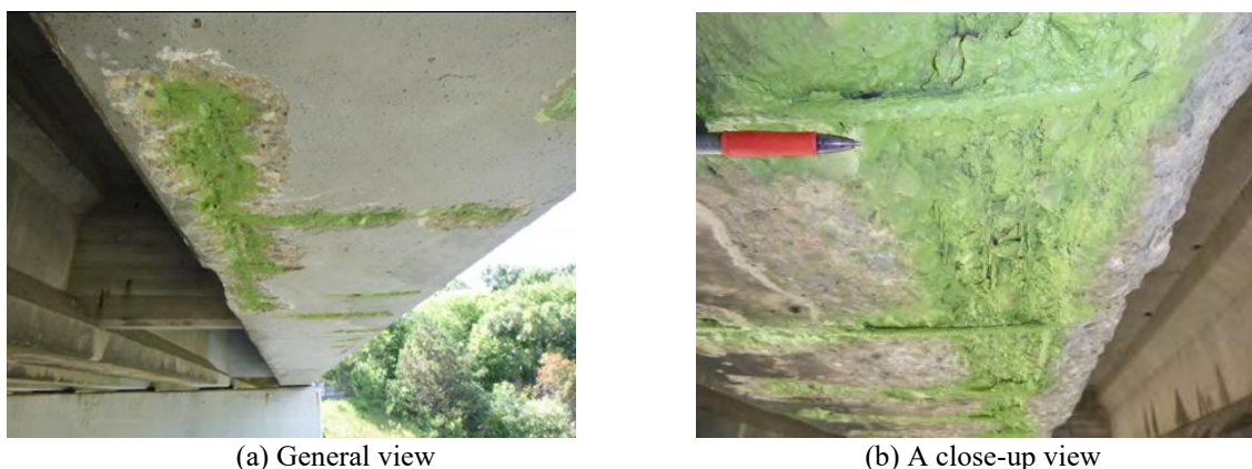
Figure 6-8. Cleaning and coating of exposed steel at the beam soffit.
