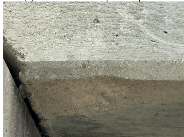
(d) South fascia beam in span 2w at pier 1w, overcast cracking
