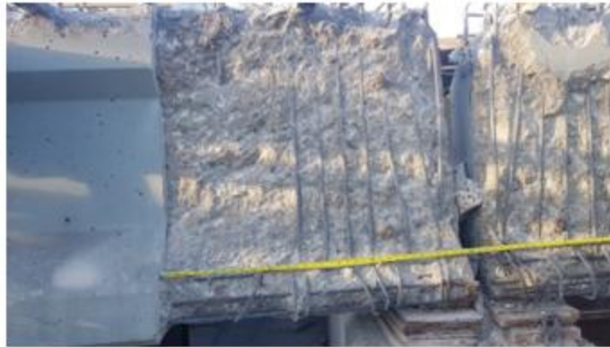
(c) Chipped out and cleaned beam ends
