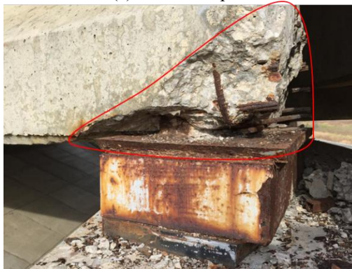
(c) Severe spall
