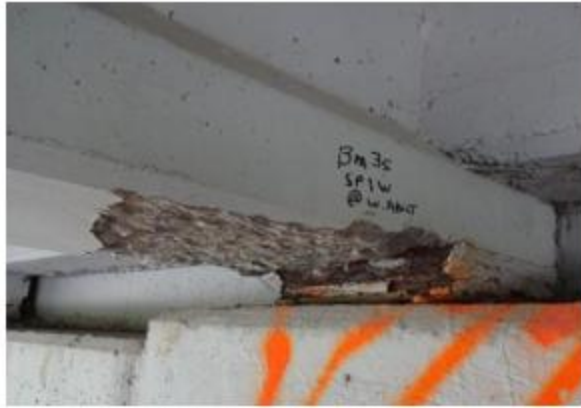
(a) Bottom flange soffit
