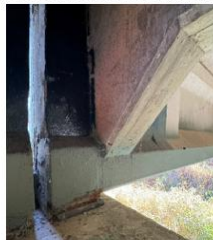
(e) Beam end with partial-height repair, FRP, and CSC
