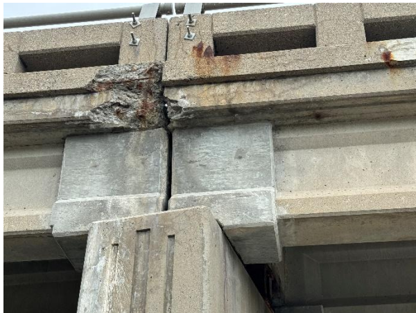
(a) South fascia beam end repairs at pier 1w
