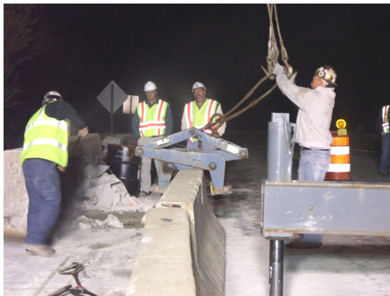
Figure 5-65. Removal of safety barriers
