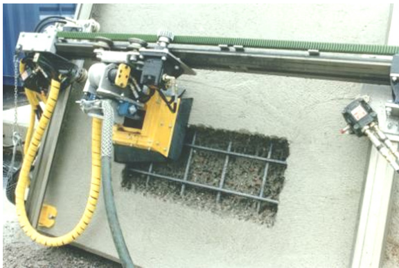
(a) Concrete removal by hydrodemolition (Source: http://nationalhydroinc.com )
