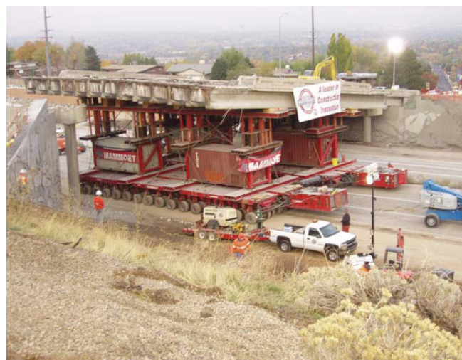
Figure 2–11. Removal of the bridge using SPMT system (Source: Ardani et al. 2009)
