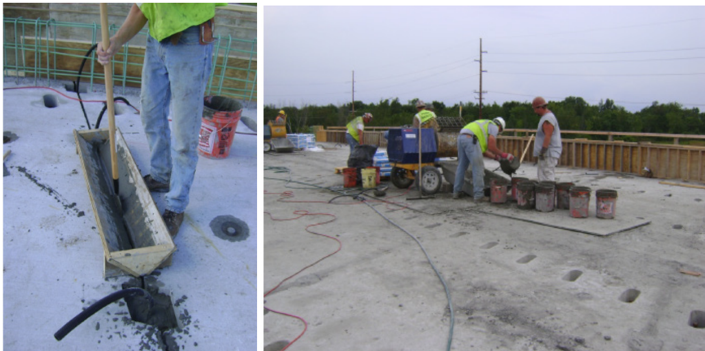
Figure 2-8. Grouting of full-depth deck panel connections (Source: Courtesy of MDOT)
