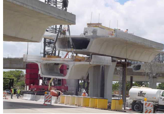
(b) A saw cut section of a segmental bridge (Source: Lwin 2003)
