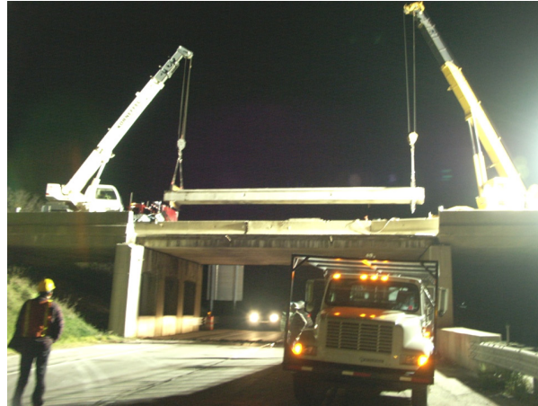
Figure 5-63. Removal of a box-beam
