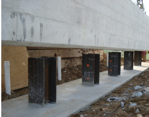
Figure 5-17. Concrete slab on ground to maintain the proper grade for placing the abutment stem (Source: Photo courtesy of MDOT)
