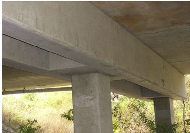
Figure 5-24. Precast bent cap with cavities (Source: Culmo 2009)
