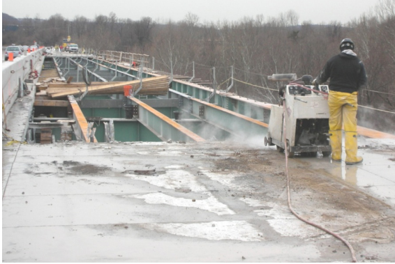
(a) Saw cutting of a bridge deck (Source: http://www.476blueroute.com )
