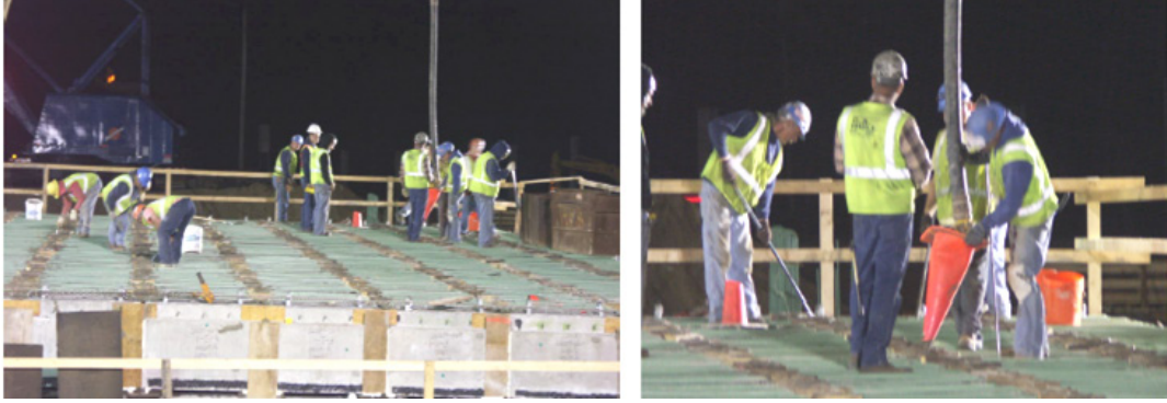
Figure 2-6. Grouting adjacent box-beam shear keys using type R-2 grout (Oakland Drive over I-94, MI)
