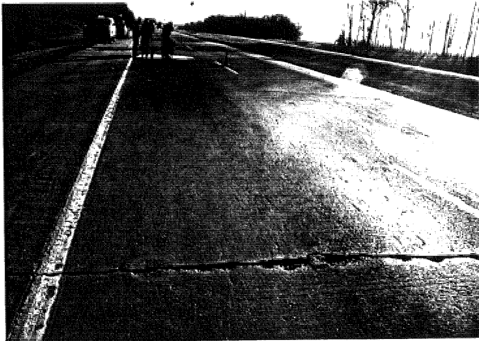
Overview of section MI1-3, showing a spalled sympathy crack in the foreground. The terrain is relatively level in this test section.
