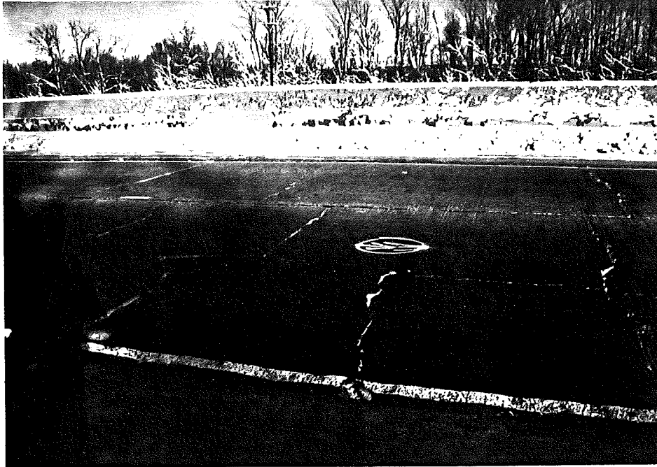
Photo #12: Pavement in the East bound test section (MI2-2). Notice the shattered slab and the spalling at the cracks.
