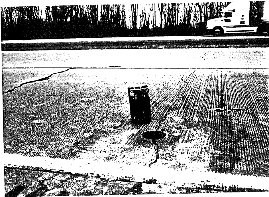
This photo shows two cracks of different severities in section MI1-2. Spalled and faulted cracks are common to this pavement section, though as seen here, some less severe cracks are also present. The more severe crack in this photo is a sympathy crack, while the other is not.
