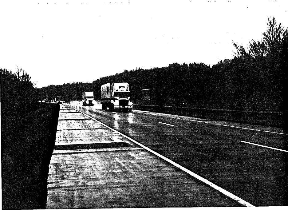
Overview of section MI2-1. This section (west bound) is on a gentle fill slope. The pavement is in excellent condition, with only two minor cracks found in the test section.
