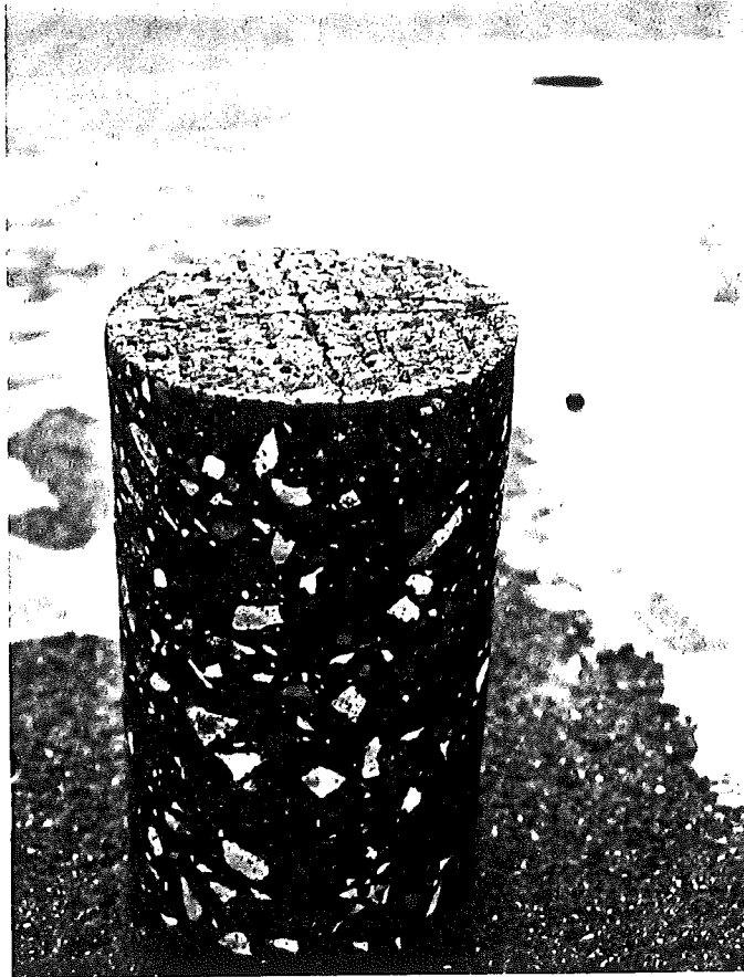
Close-up view of a cored sample in section MI-2 showing a shrinkage crack. The crack follows the tining pattern in the pavement, and extends approximately one inch deep into the concrete. This section contains recycled concrete.
