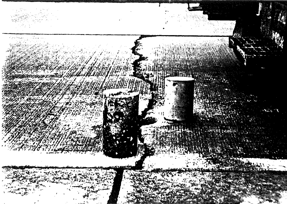
Photo #2: Typical crack in section MI1-2, recycled concrete on open-graded drainage course.
