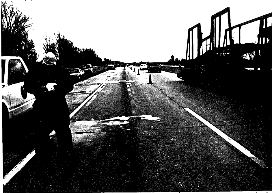
Overview of section MI1-4. This, as all sections of the Lawrence project, is on relatively level ground, with little cut or fill necessary. An intact transverse joint is visible in the foreground.
