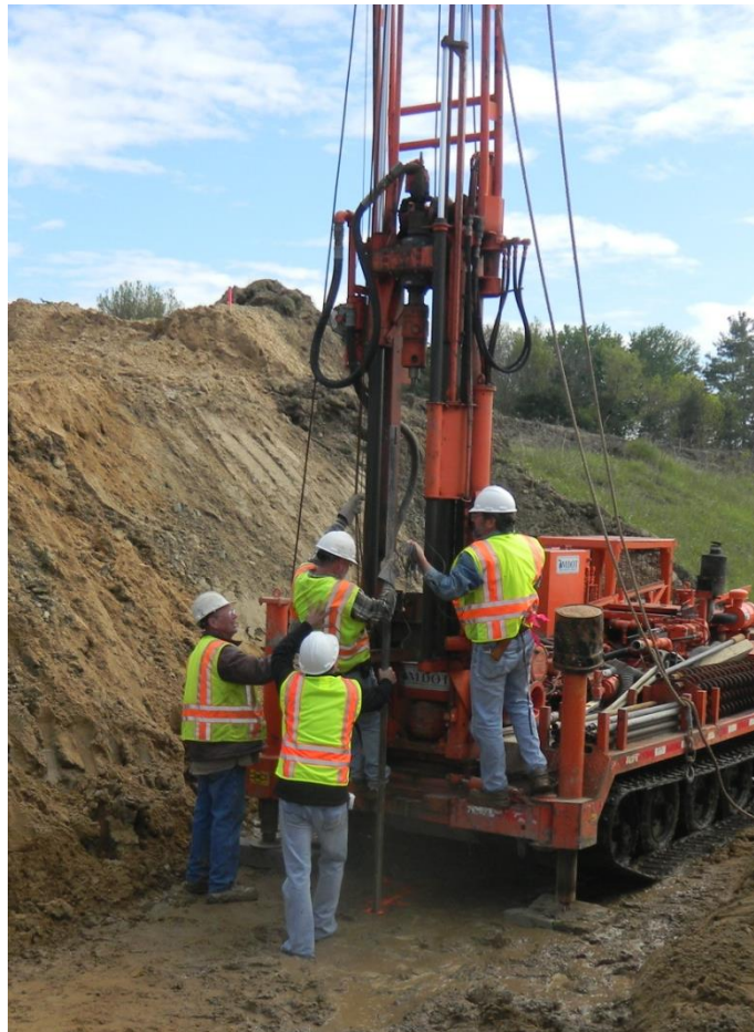
Figure 2-9 Installation of embedded sensors
