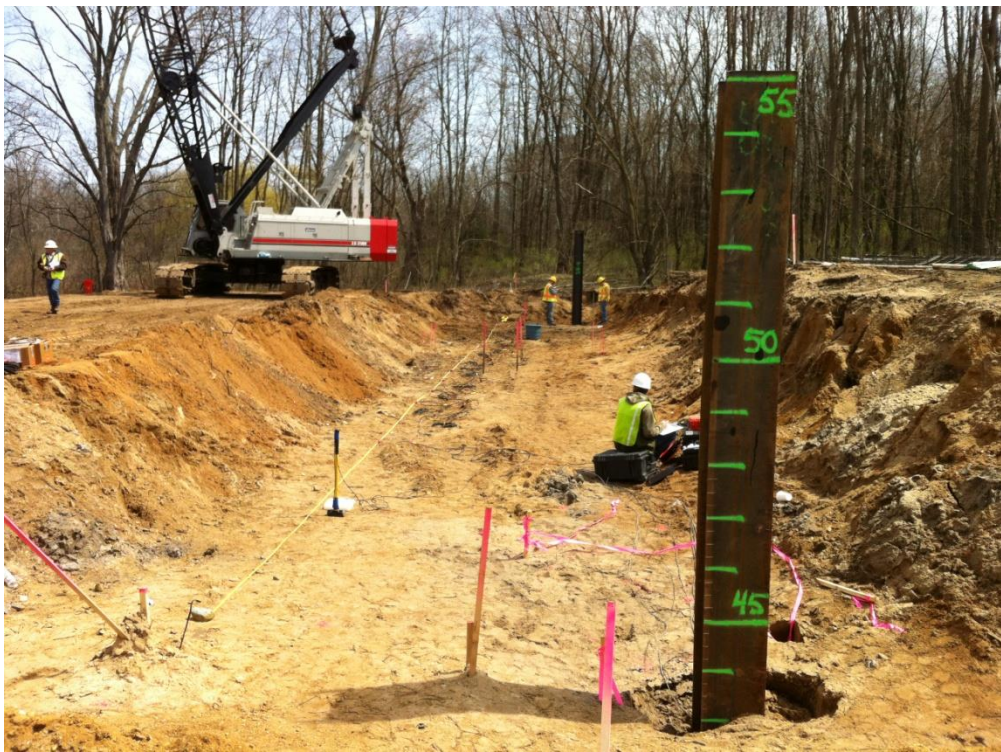
Figure 2-27 Test piles #1 & #18 after the end of driving at US-131 A site
