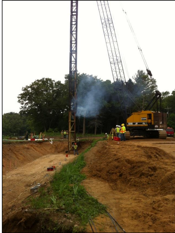
Figure 2-31 Driving test pile #37 at US-131 B site
