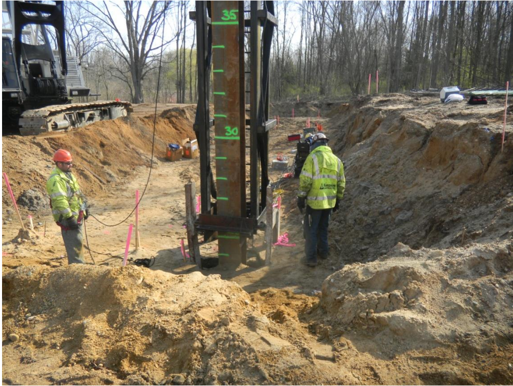
Figure 2-26 Driving test pile #1 at US-131 A site
