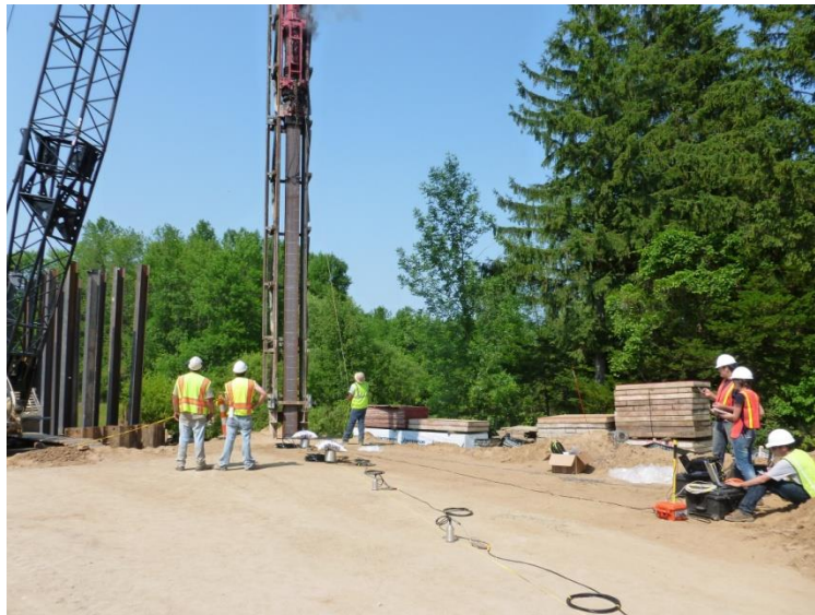
Figure 2-12 Pile driving at M-25 site
