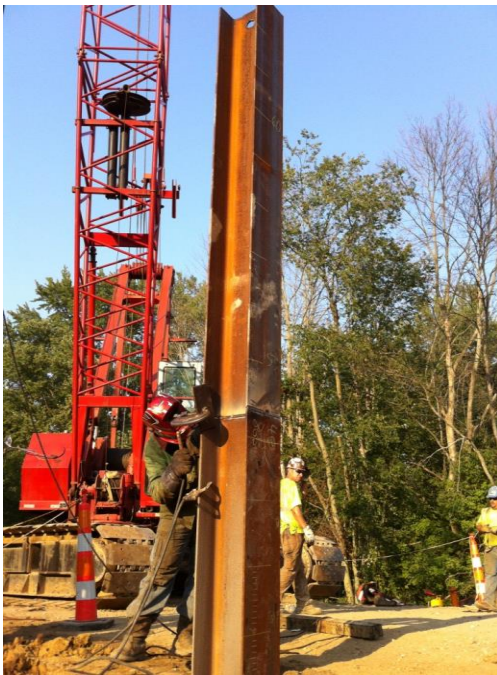
Figure 2-16 Welding second section of pile
