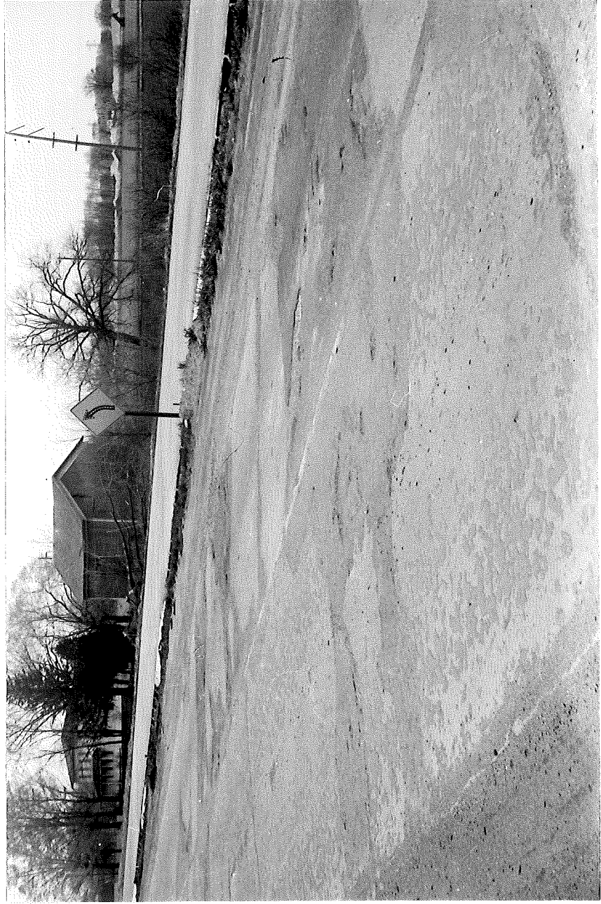
Figure 5. Example of type of old surfacing that was capped as F-88-54-C4.
