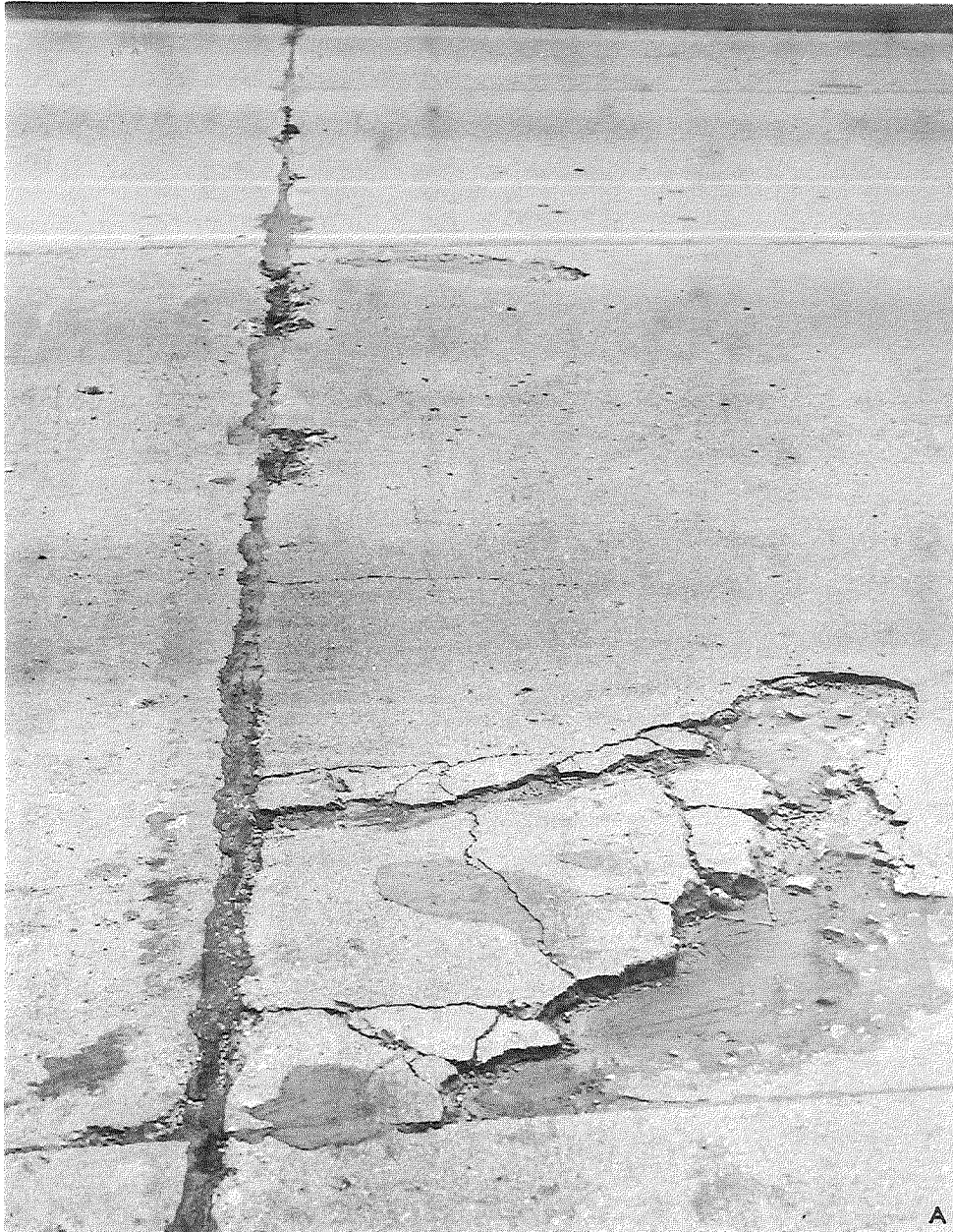
Figure 3. "Joint 2" is shown in an overall view (A). During cleaning for inspection and repair, dowel misalignment (upward tilt) on the morning side of the joint, was clearly visible (B, C). Webster Ave. at Fifth St.
