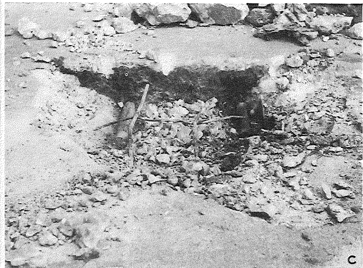
Figure 3. "Joint 2" is shown in an overall view (A). During cleaning for inspection and repair, dowel misalignment (upward tilt) on the morning side of the joint, was clearly visible (B, C). Webster Ave. at Fifth St.
