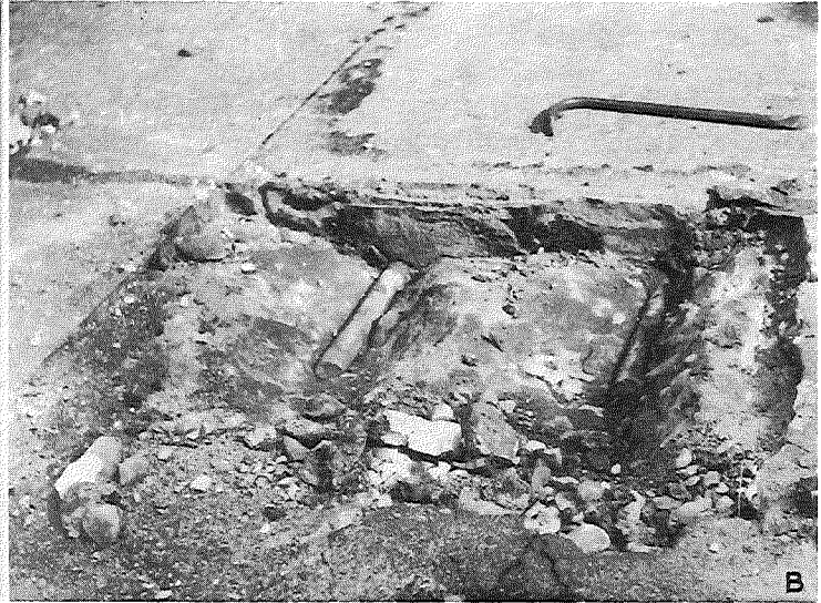
Figure 3. "Joint 2" is shown in an overall view (A). During cleaning for inspection and repair, dowel misalignment (upward tilt) on the morning side of the joint, was clearly visible (B, C). Webster Ave. at Fifth St.
