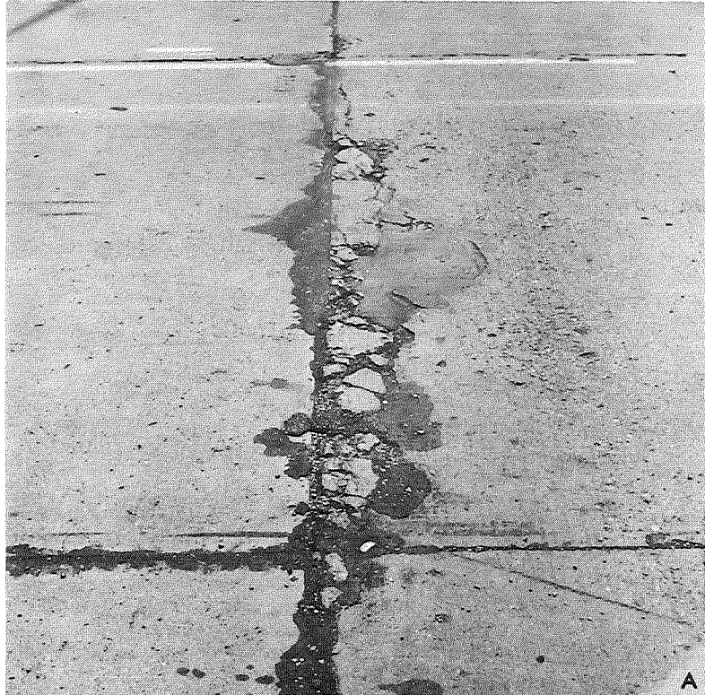
Figure 4. "Joint 3" where opening had occurred about 6 in. on the spalled side of the joint groove, is shown in an overall view (A). In the spalled area, reinforcement was embedded only 7/8- to 1 in. beneath the concrete surface (B). The reinforcing mat here was found to have been placed crosswise at the time of construction (C). A No. 4 gage wire was found to have broken within the slab, probably soon after construction (D, E), indicating that the pavement was opening at this point rather than at the joint. Muskegon Ave. at Ninth St.
