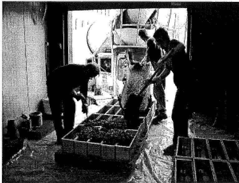
Photo 11-3. Placing concrete on the Dillman Hall loading dock
