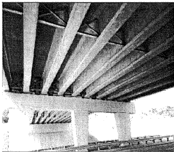
Figure 10-50. Steel Diaphragms between the Beams and the Cross-Section
