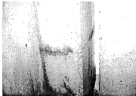
Photo 6-8. Condition State 8—Moderate Cracks with efflorescence, water-stains, and/or corrosion (a) E2-S3-E-B from 25132 S34 and (b) E2-S8-E-S.2 from 41029 S16-4
