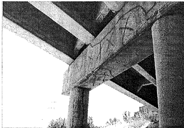
Photo 3-38. Condition of pier and pier cap
