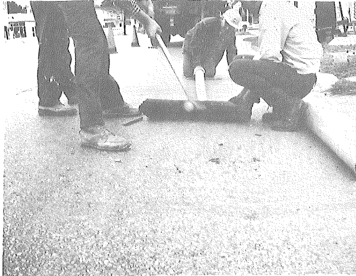
WAY OF DRIVING SECTIONS ONE ONTO THE OTHER.
