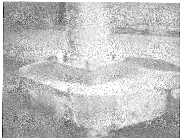
FINISHED BASE OF CANTILEVER AFTER ERECTION WAS COMPLETED.
