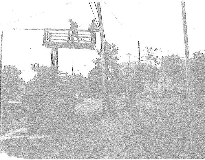
BOLTING OF ARM ON SHAFT.
