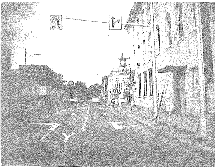
SECTIONAL POLE CANTILEVER ON M-155 @ BL-96 (GRAND RIVER AVE.), CITY OF HOWELL. DATE OF ERECTION: 9-8-69.
