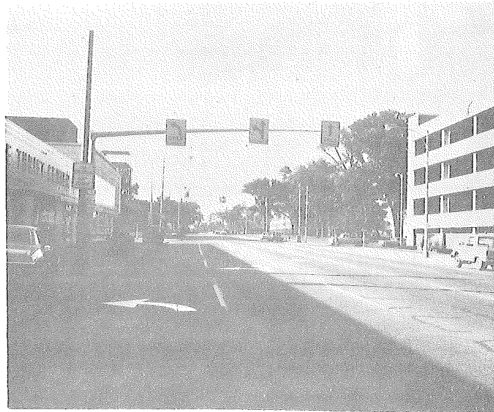
SECTIONAL CANTILEVER SUPPORTING LANE CONTROL SIGNS FOR THREE LANES OF OPERATION ON CAPITOL AVE. AT KALAMAZOO STREET, CITY OF LANSING.
