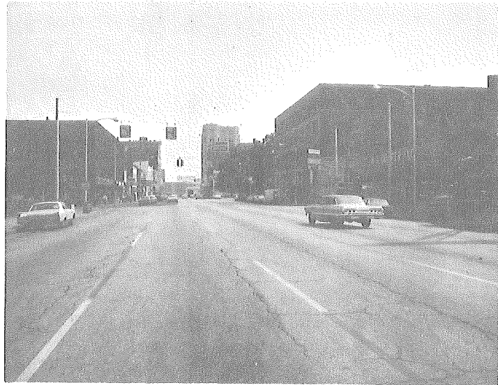
TWO STEEL POLES WITH SPAN WIRES INSTALLATION SUPPORTING LANE ASSIGNMENT SIGNS ON US-131 BR, BL-94, M-43 (MICHIGAN AVE.) @ US-131 BR (PARK ST.), CITY OF KALAMAZOO.
