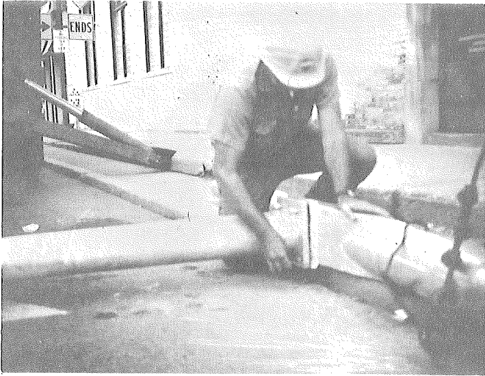
BOLTING ARM ON SHAFT OF CANTILEVER.
