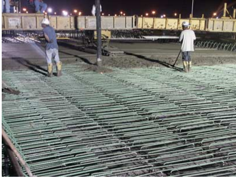
Photo 5-3. Concrete placement of Vreeland over I-75
