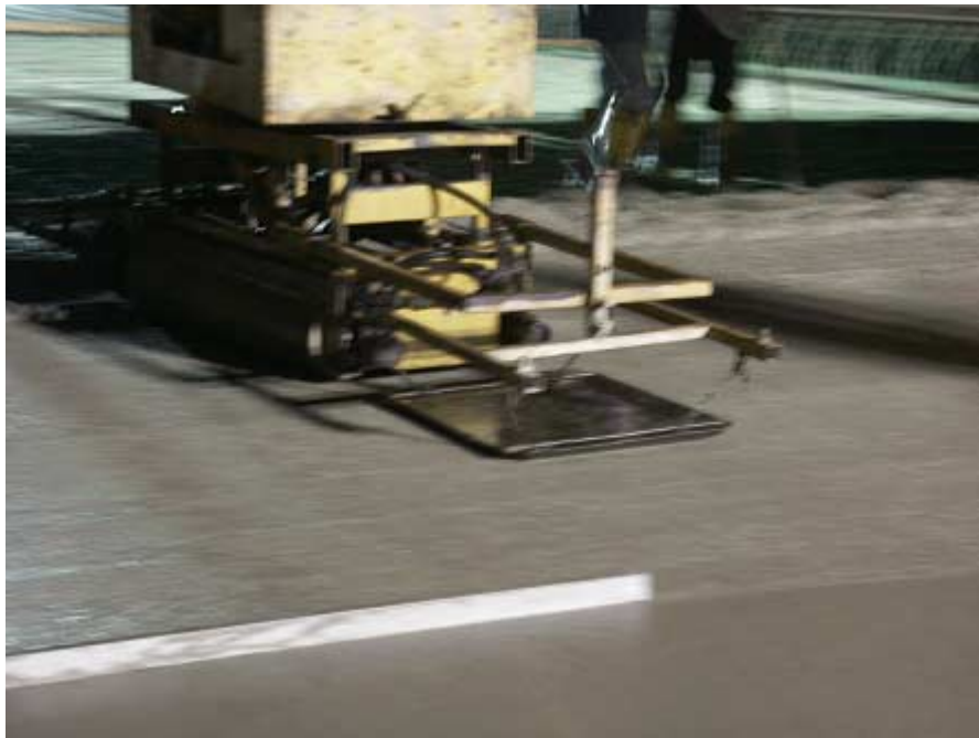
Photo 5-5. Finishing concrete of Vreeland over I-75
