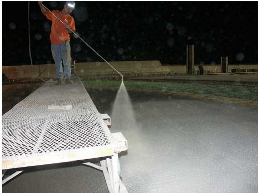
Photo 5-8. Application of curing compound of I-94 over Quinn road
