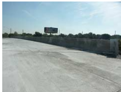
Photo 5-9. Diamond ground deck surface of bridge S06 of 82194
