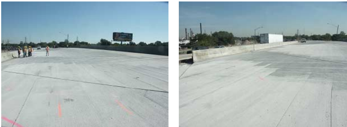
Photo 5-10. Replaced deck of bridge S06 of 82194
