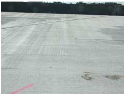
Photo 5-9. Diamond ground deck surface of bridge S06 of 82194
