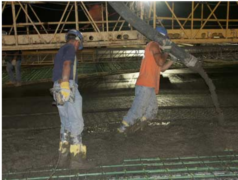
Photo 5-2. Concrete placement of I-94 over Quinn road
