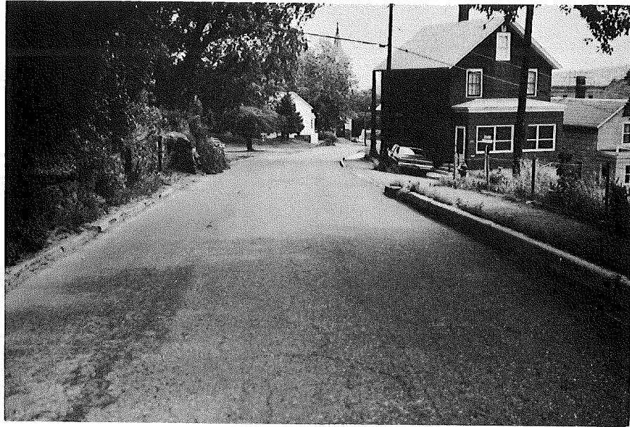
SOUTHEASTBOUND WHITE STREET
