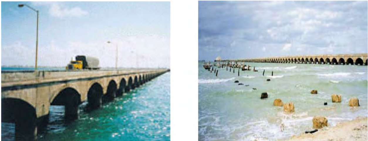
Figure 1. Pier in Progreso, Yucatan Peninsula, Mexico, constructed in 1937-41 with equivalent type 304 stainless reinforcement. Pictures dated December 1998. Note in foreground of the right picture the remains of an adjacent pier constructed with carbon steel in the 1960's.
