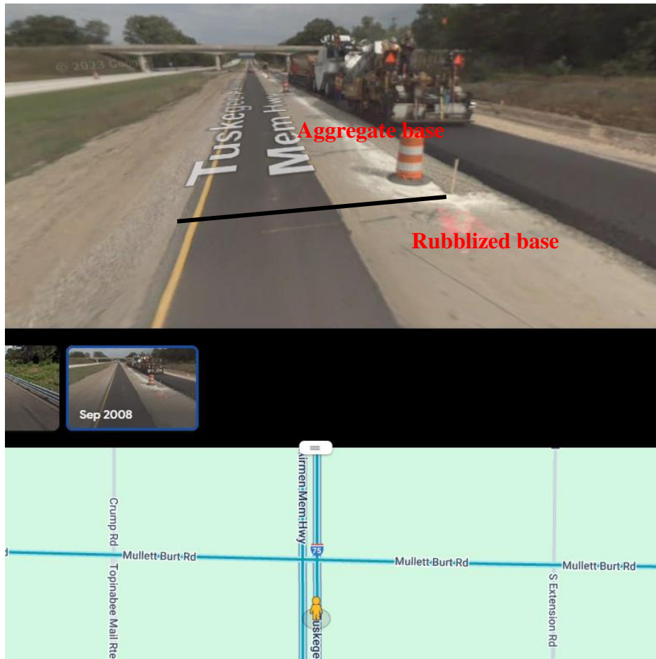
Figure 7. Construction around Sta 601+00 in September 2008 from Google Maps
