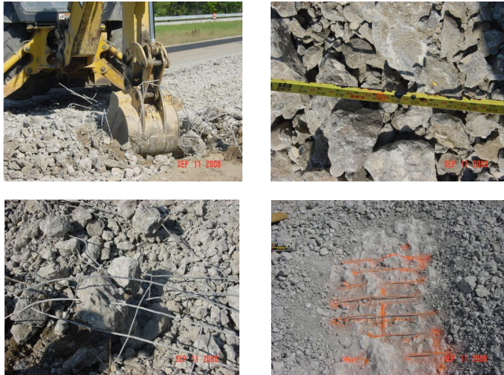
Figure 8. Field rubblization process for the I-75 NB project
