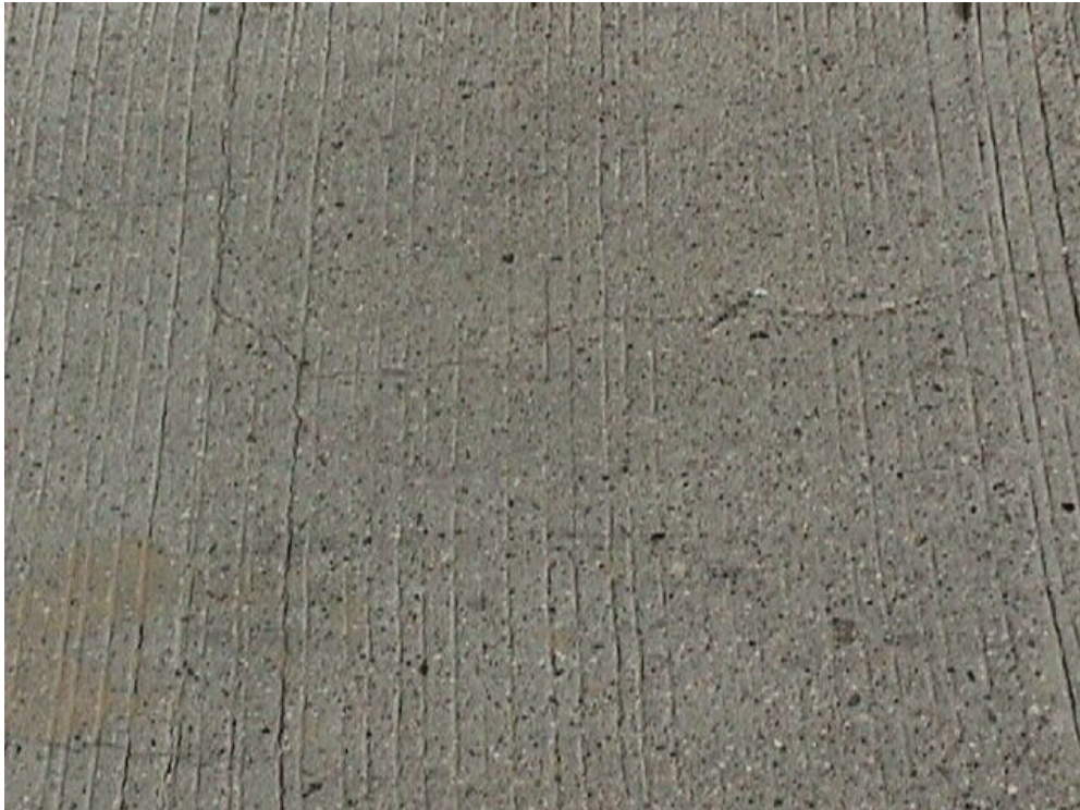
Figure 3-5. Shrinkage cracks
