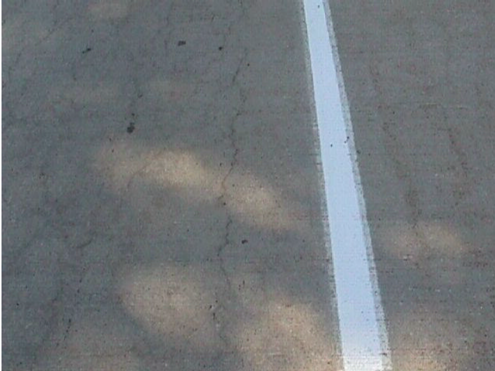
Figure 3-6. Longitudinal cracks (top of the deck)
