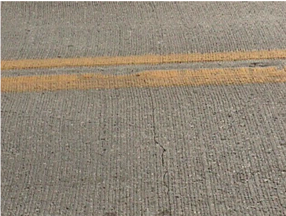
Figure 3-9. Transversal cracks
