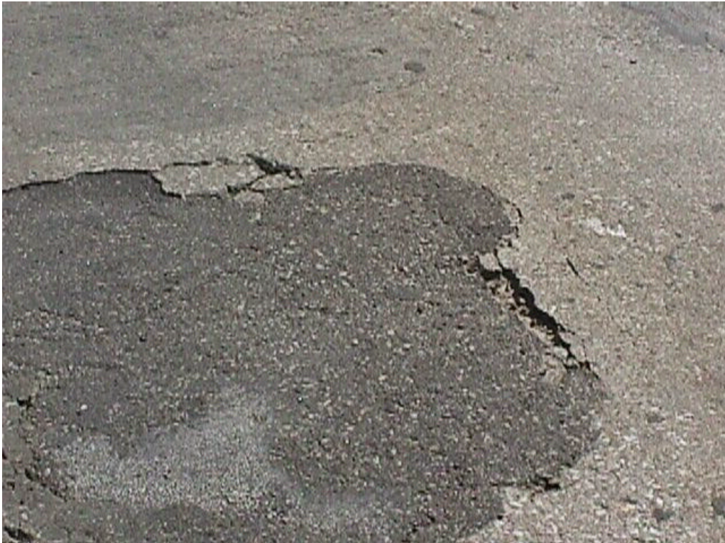
Figure 3-15. Delamination
