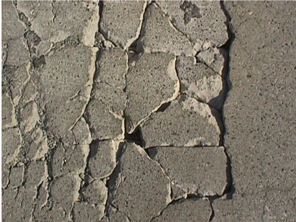
Figure 3-18. Disintegration
