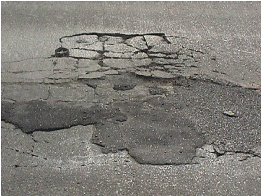
Figure 3-17. Delamination
