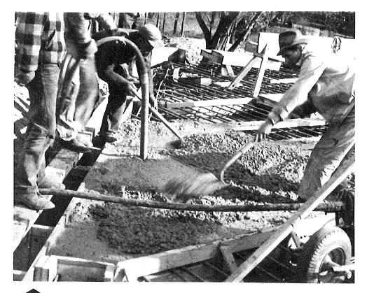
VIBRATION OF CONCRETE IN FORMS PARTIALLY FILLED. NOTE SOUPY CONCRETE APPEARING AROUND VIBRATOR. SS BI OF 33-7-9, 4
