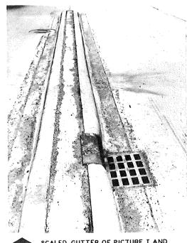
SCALED GUTTER OF PICTURE I AND ADJACENT UNSCALED SLAB, GRAVEL AGGREGATE, ROAD SECTION, CORE L, 2.97 % AIR. L
