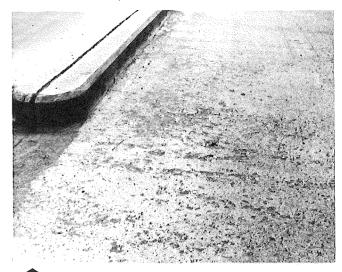
SCALED SLAB, POUR B, CORE B, 1.96 % AIR. B STATION II + 20 - 5 FT. RT. OF CENTER.
