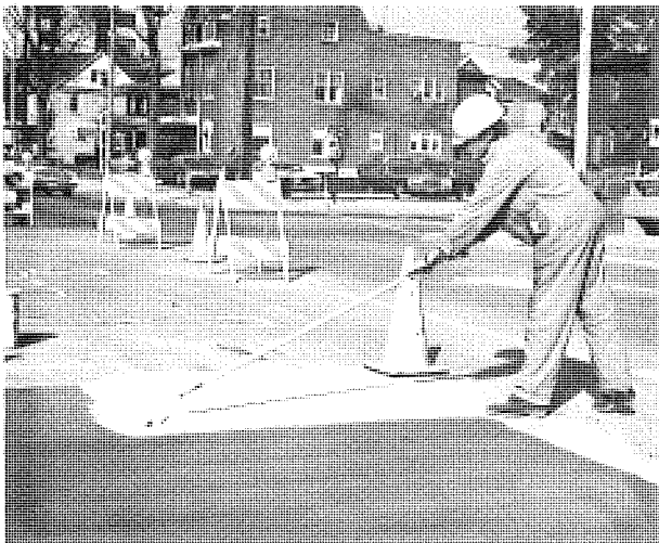
Surface is screeded, floated, and troweled. Crown curvature was cut into the screed board. ▶
