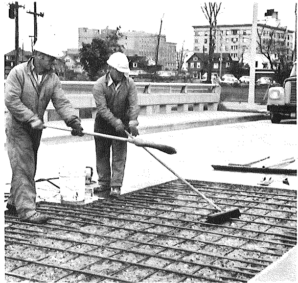
◀ When consolidating the low slump Em-beco 411A mortar, the vibrator is pulled between rebar locations to free any air entrapped beneath the bars and completely surround the bars with concrete (note the initial priming mortar).
