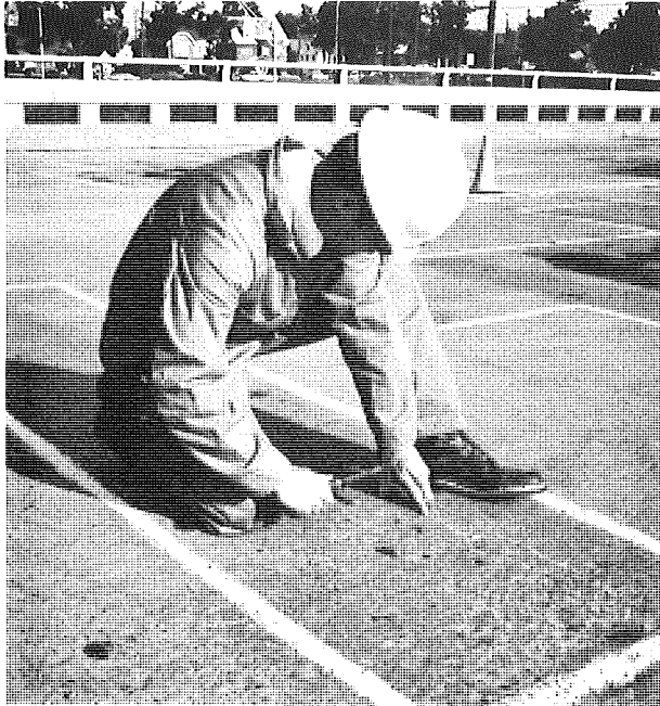
Locating position of reinforcing bars in delaminated area. ▶
