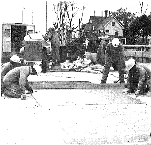
◀ A white membrane curing compound was applied three hours after brooming.
