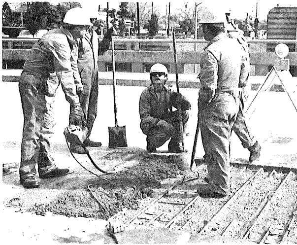
Surface is screeded, floated, and troweled. Crown curvature was cut into the screed board. ▶
