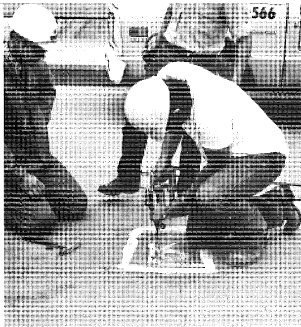
A vacuum cleaner is used to remove drill dust from around ports. ▶
