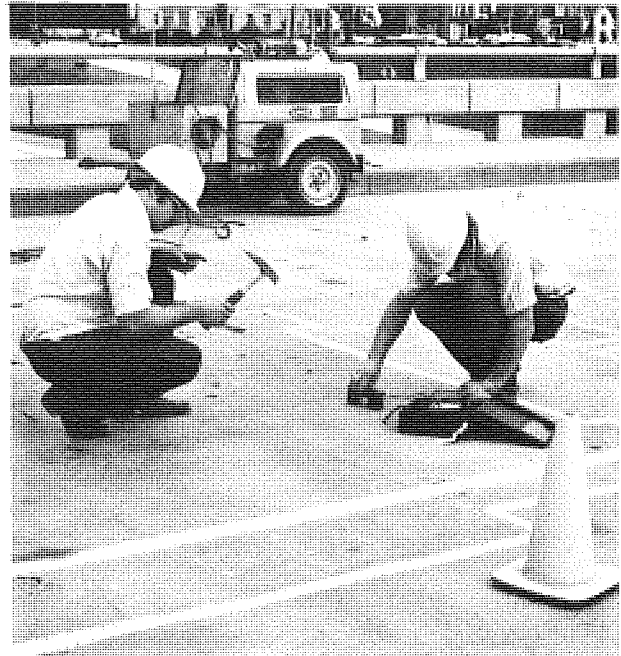
◀ Three-eighths in. holes are drilled for injection and vent ports.
