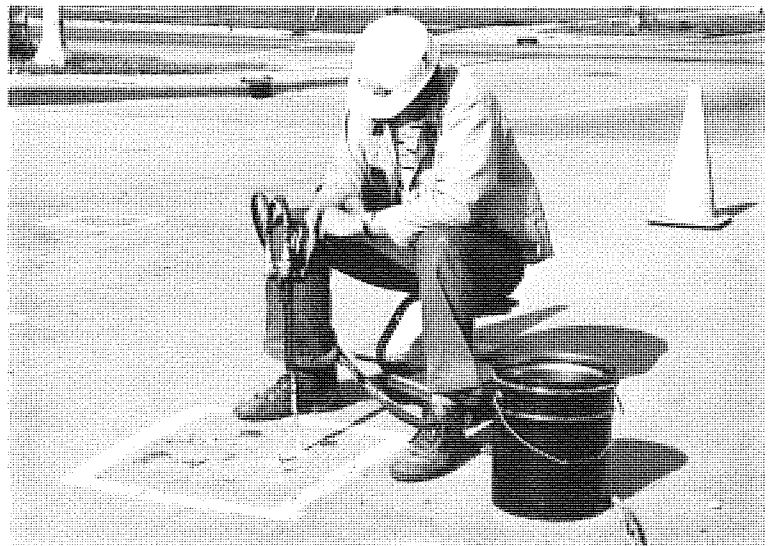
Figure 6 (Cont.). Sequence of operations for epoxy grouting procedure.
