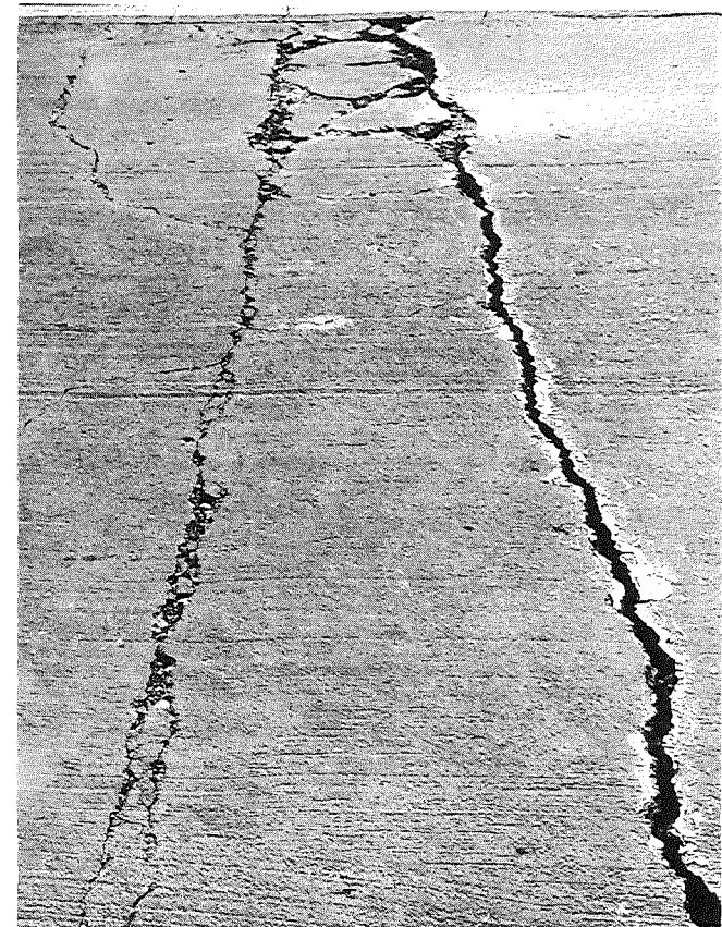
Figure 3. Failure and proposed repair at Sta 990+82 eastbound, in conventional concrete pavement. Photographed from traffic lane shoulder.
