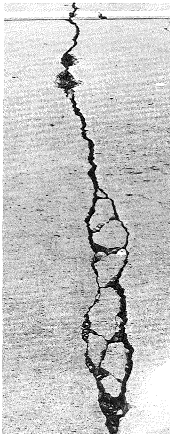
Figure 1. Failure and proposed repair at Sta 1045+40 westbound, in continuously reinforced wire mesh pavement. Photographed from traffic lane shoulder.
