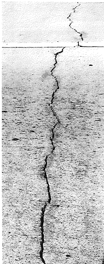
Figure 3. Failure and proposed repair at Sta 990+82 eastbound, in conventional concrete pavement. Photographed from traffic lane shoulder.
