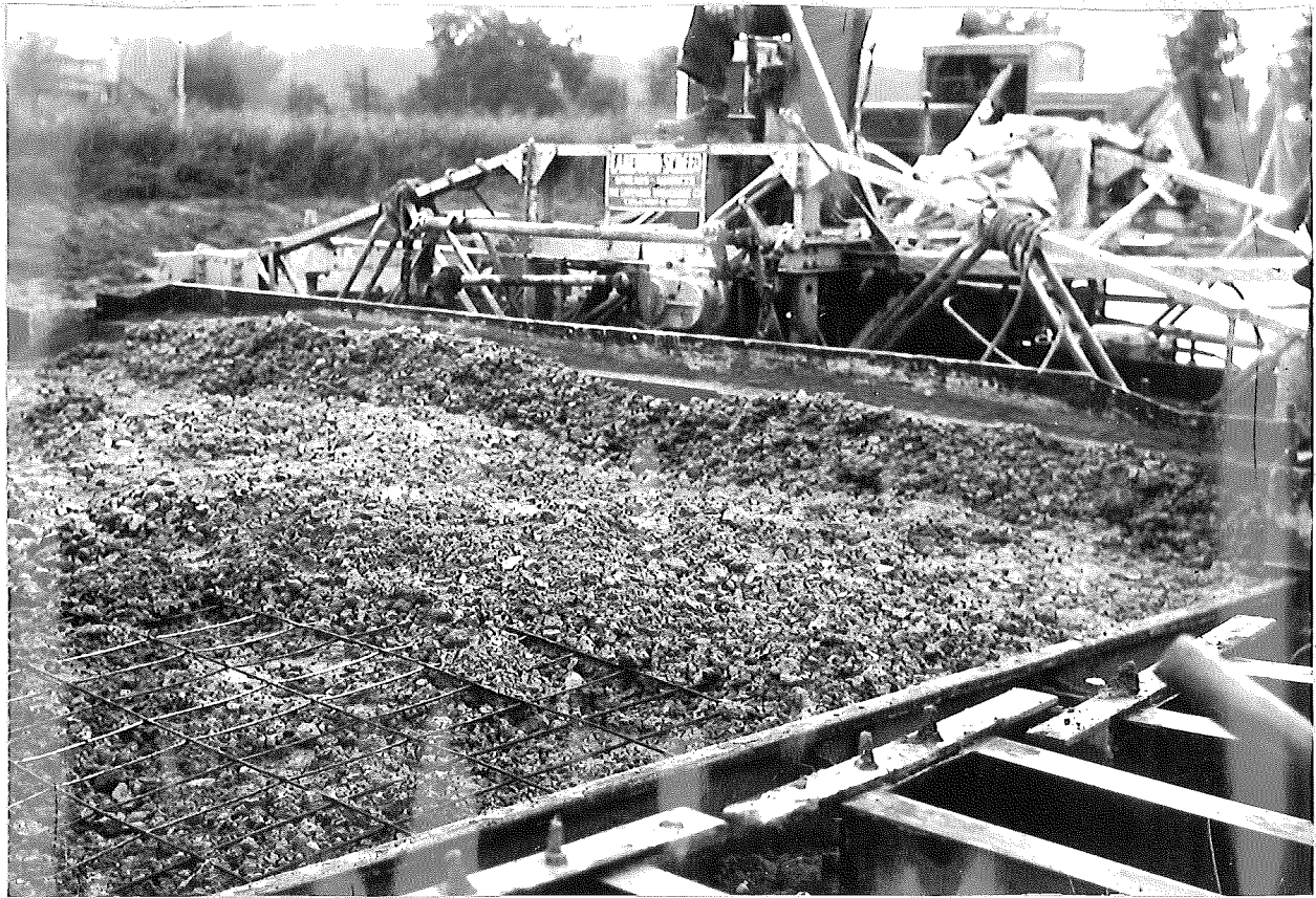
Lakewood Vibratory Screed used on Projects 19-27 and 33-21 Spreading concrete, first run
