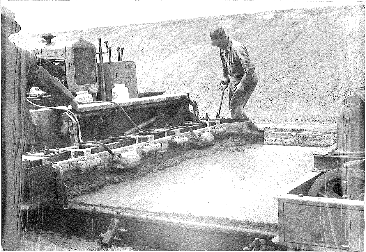
Vibrating screed on finishing machine, Project 41-34, 06
