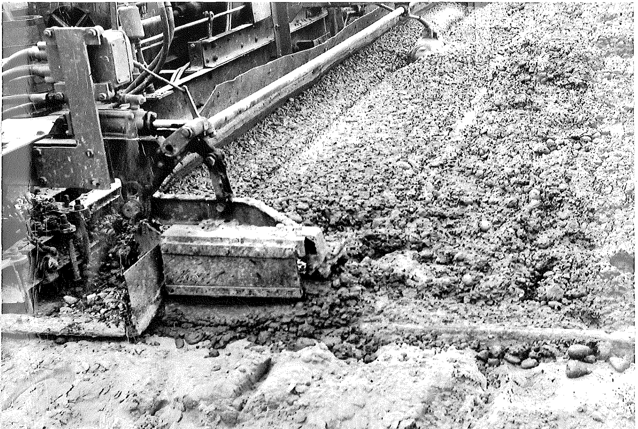
Vibratory Tube in operation
