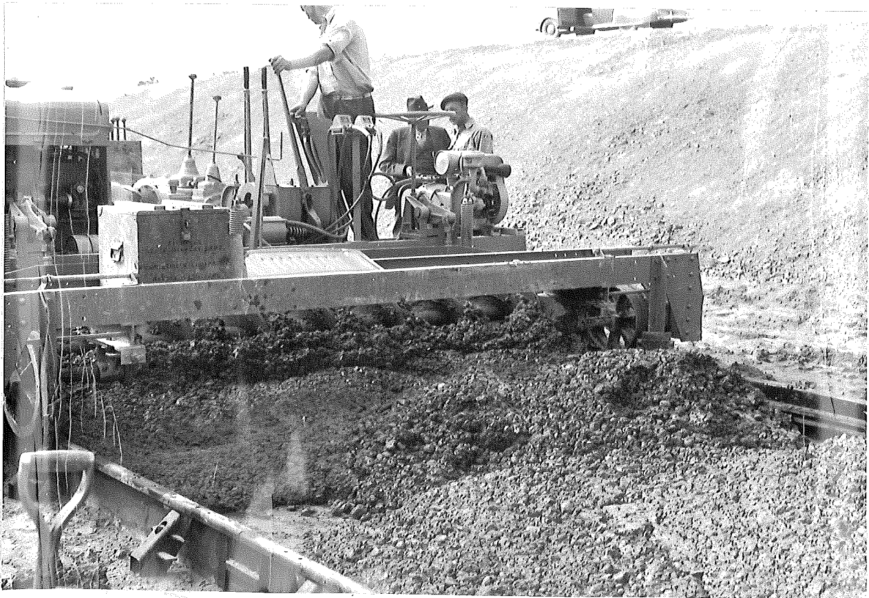
Jaeger Screw-type Spreader with a plank vibratory strike-off. Project 41-34, 06
