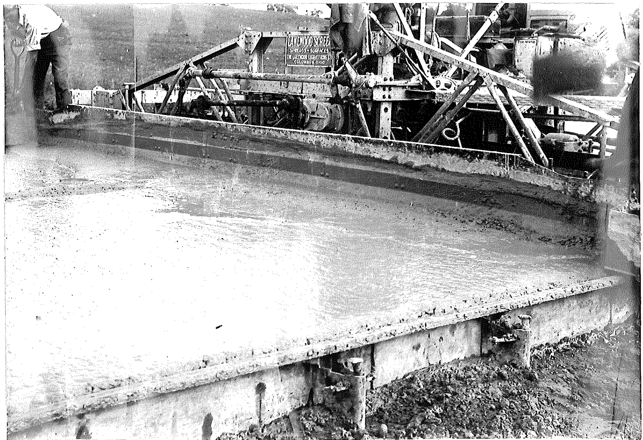
Lakewood Vibratory Screed, final run
