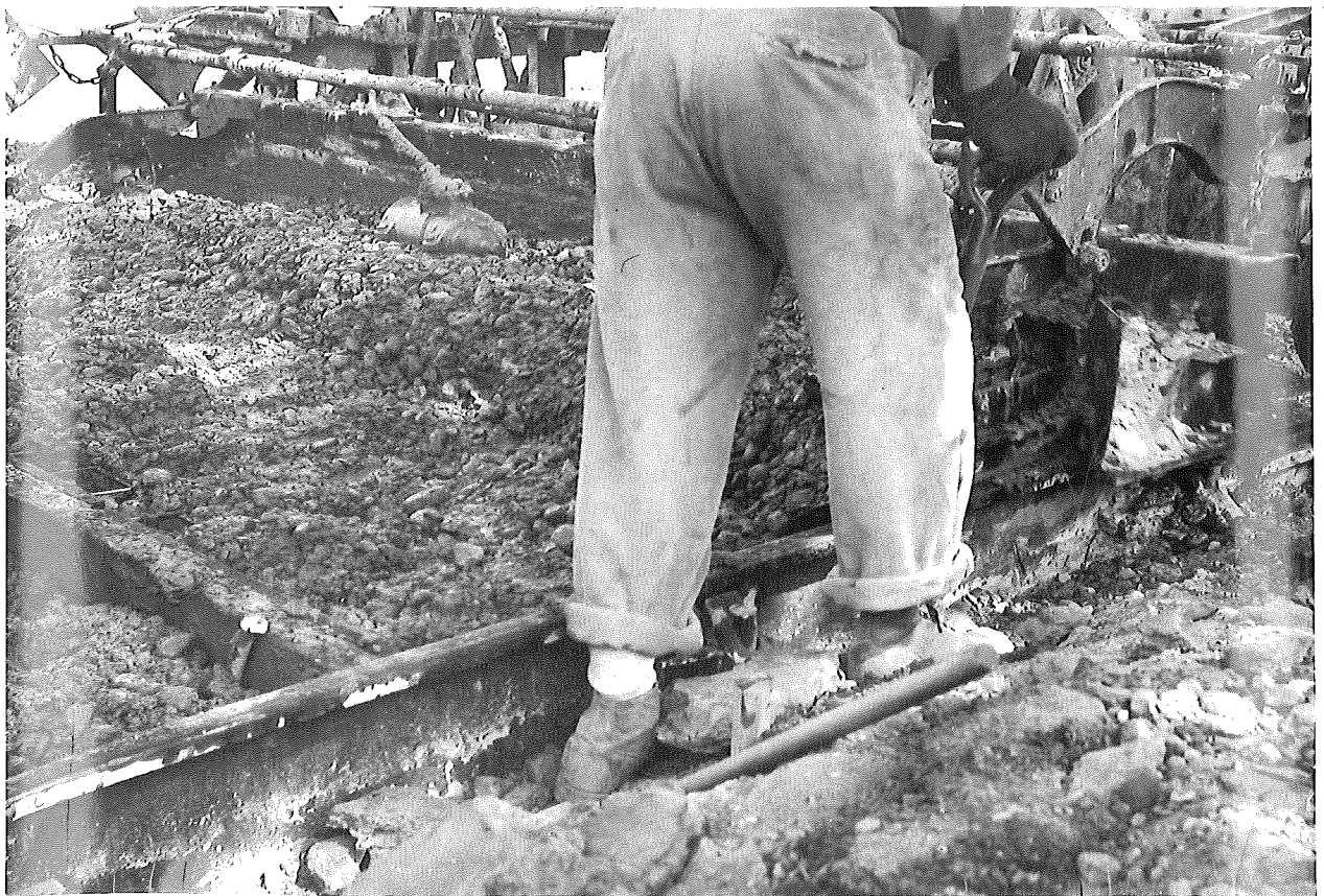
Vibratory tube in operation, Projects 33-39 and 19-3
