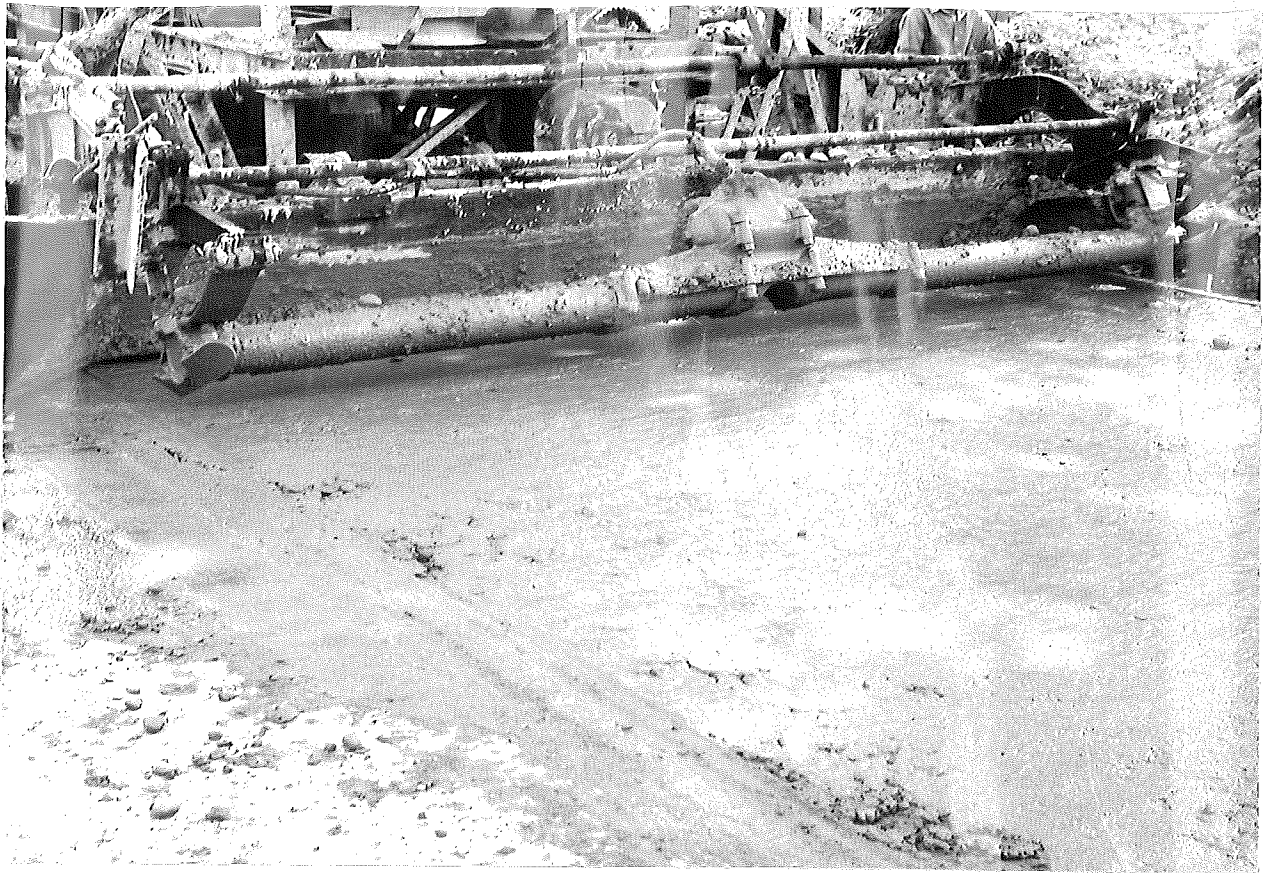
Eleven-foot Jackson Vibratory Tube used on Projects 33-39 and 19-3
