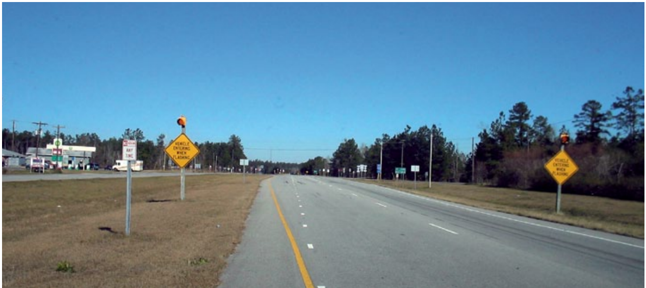
Figure 2: Through Vehicle Activated Warning Sign System in North Carolina Photo courtesy of NCDOT
