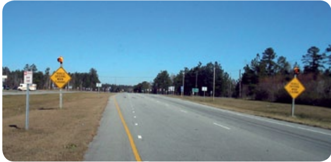
North Carolina, double sign Photo courtesy of NCDOT
