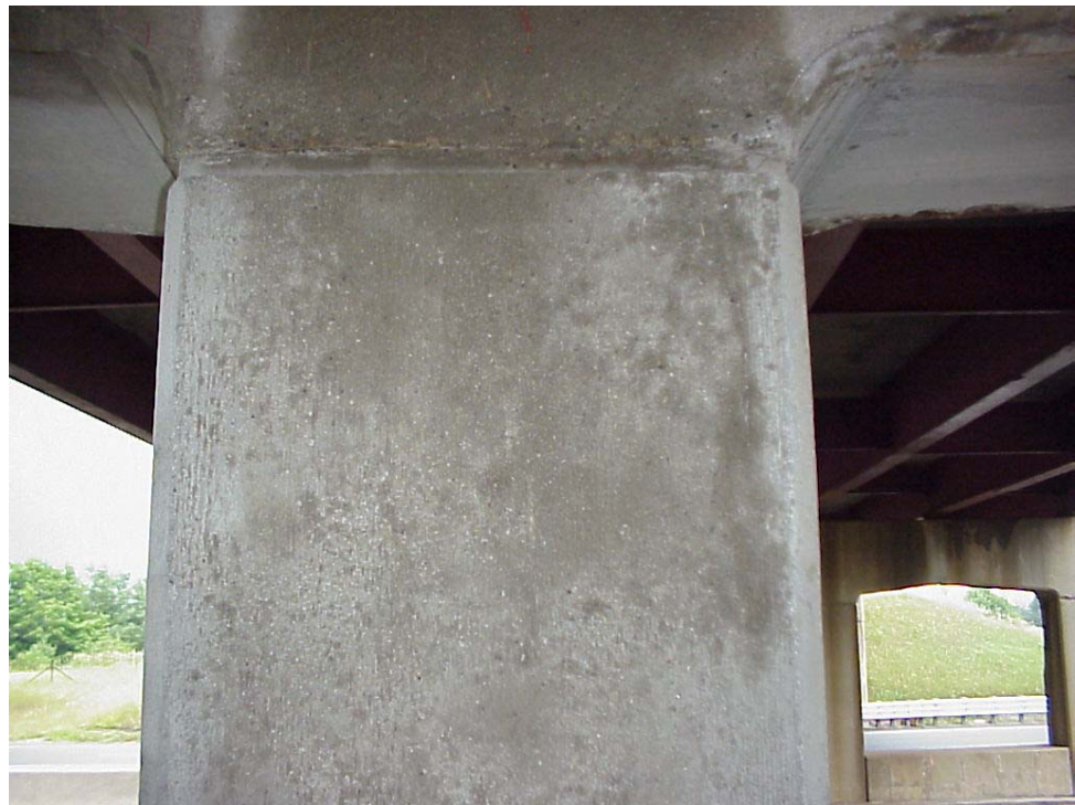
Figs. 5.2 Column condition after surface repairs
