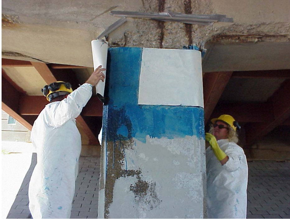
Fig. 5.5 Field installation of carbon wrap to selected columns
