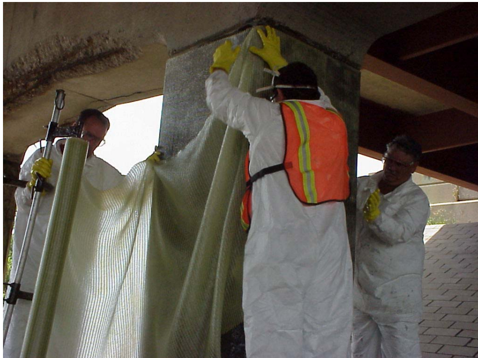
Fig. 5.4 Field installation of glass wrap to selected columns
