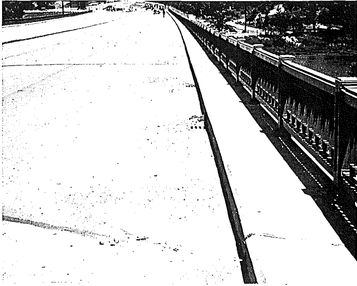
FIGURE 7. DEEP AND PROGRESSIVE SCALING AROUND CATCH BASIN ON SPAN 3, OUTSIDE NORTHBOUND LANE.
