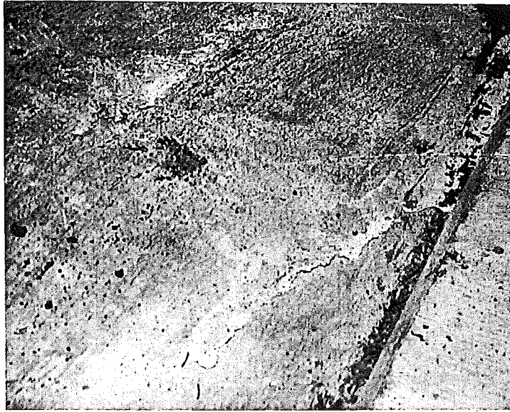
FIGURE 3. TYPICAL VIEW OF PITTING ON SPAN 2 ON NORTHBOUND LANE CLOSEST TO MEDIAN.
