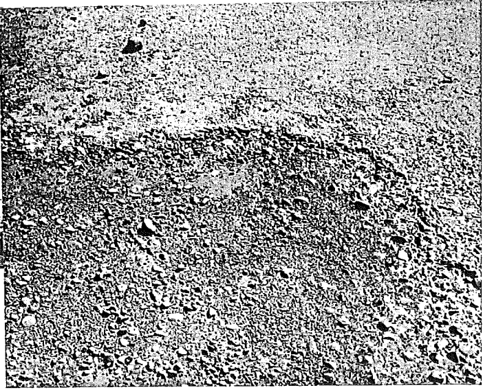
FIGURE 13. DETAILED VIEW OF SCALING SHOWN IN FIGURE 12.
