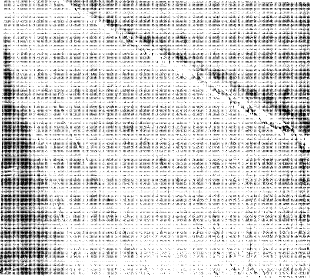
Figure 3. Typical distress conditions of the original 13-year old asphaltic concrete pavement, Construction Project Mb 72013/06140A, US 27 west of Houghton Lake.
