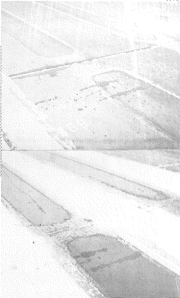
FIG. 6. CONCRETE SECTION DURING ICY CONDITION, NOTE BARE SURFACE OVER HEATING ELEMENTS, BARE AREA SAME WIDTH AS ELEMENTS - 18 INCHES. NOTE UNMELTED AREA AT JOINTS 12-12-48
