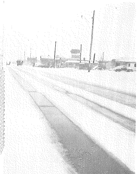
FIG.4. CONCRETE SECTION, MELTED AREAS IN FOREGROUND, SALTED AREA IN BACK AND PARALLEL.
