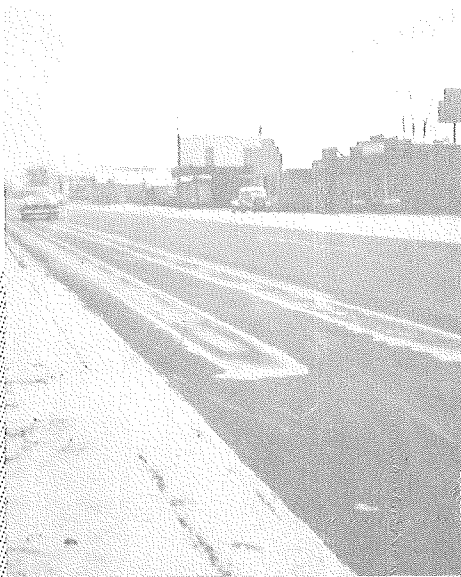
FIG.1 VIEW OF BITUMINOUS PAVEMENT DURING SLEET STORM. ICE OVER GRID AREA IS MELTED.
