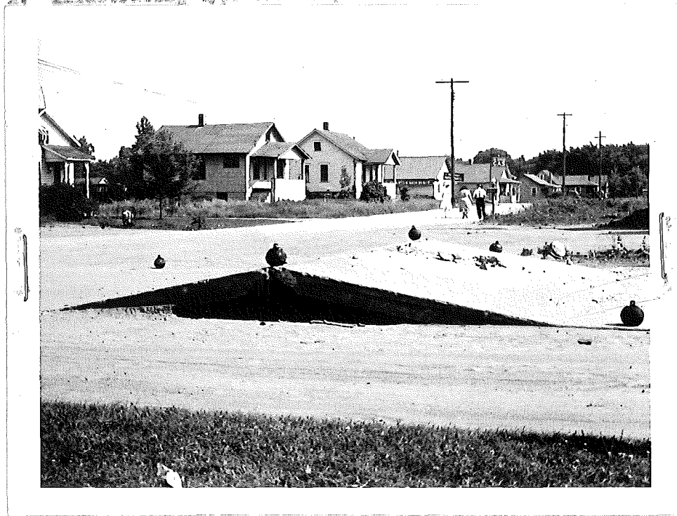
B. Illustrating type two compression failure.
