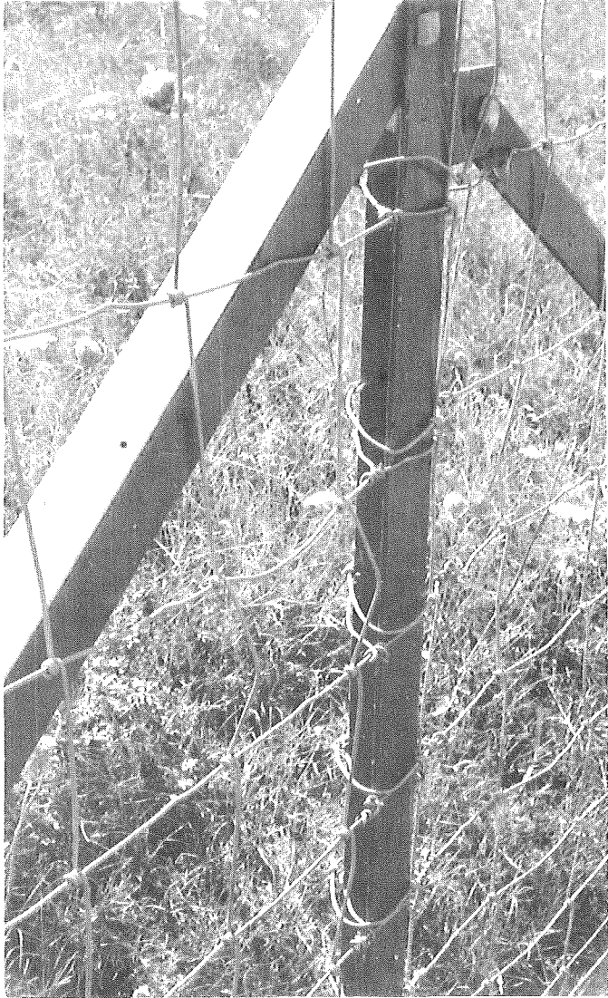
Figure 1. Splicing per MSHD specifications, tightly wrapped at post.
