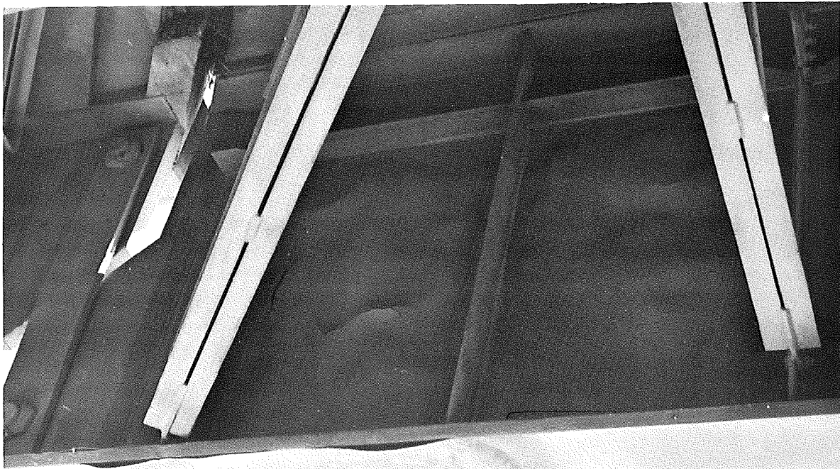
Figure 1. Beam panels on either side of bridge joint that were used in field test. Juncture of coatings is visible on bottom flanges. The boom was used for application on some areas, and for inspection.
