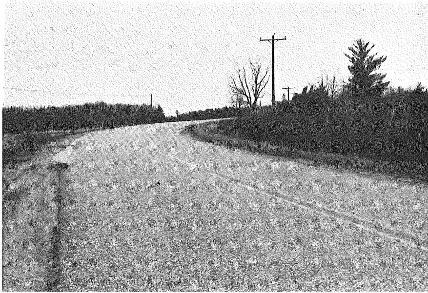
NORTHBOUND JEBAVY ROAD BETWEEN THE LINCOLN RIVER BRIDGE AND JAGGER ROAD
