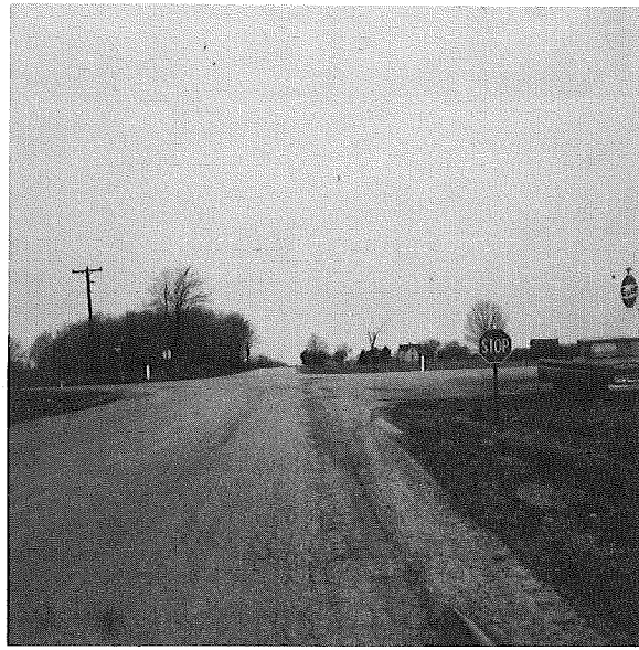
WESTBOUND SUGAR GROVE ROAD
