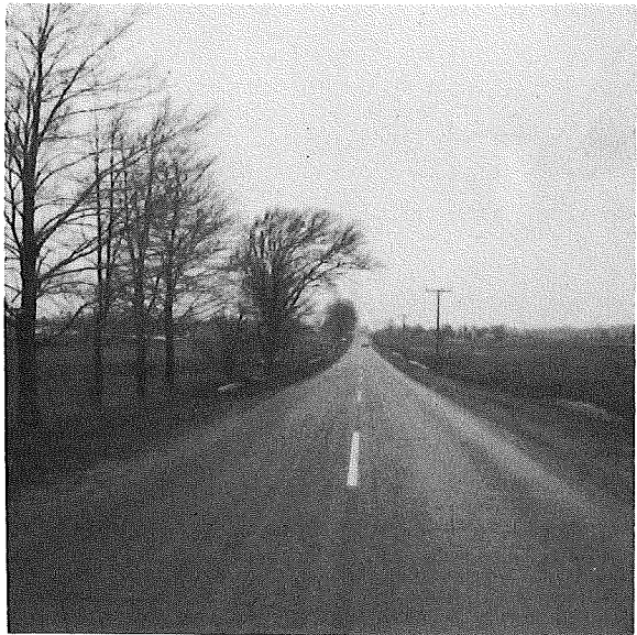
NORTHBOUND STILES ROAD
