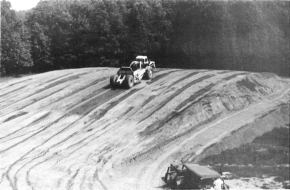
Figure 7. Surface of newly prepared stockpile showing non-uniform distribution of chloride.
