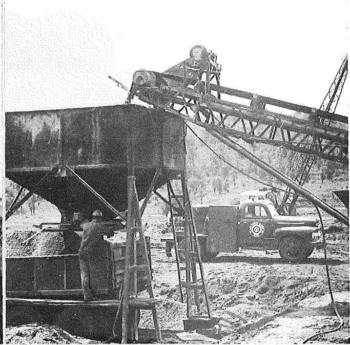
B. Belt feed to hopper. Drops to truck.
