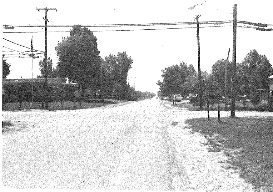
SOUTHBOUND CRYSTAL AVENUE
