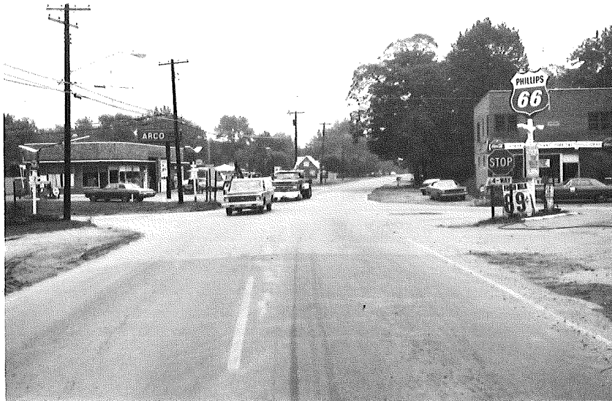
SOUTHBOUND PIPESTONE ROAD
