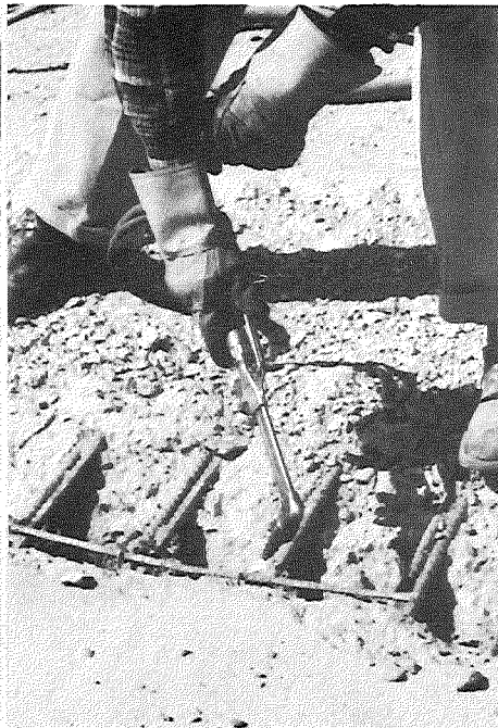
Figure 14. Cutting steel with acetylene torch.
