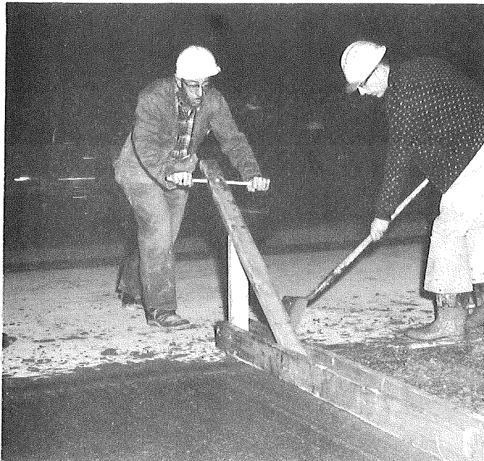
Figure 26 (bottom right). Final hand finishing of concrete surface.
