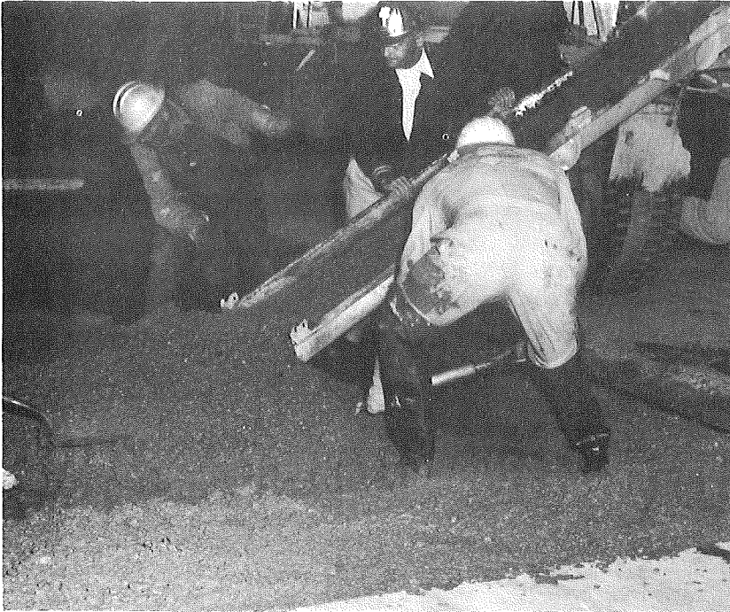
Figure 23 (top left). Delivering and spreading concrete.
