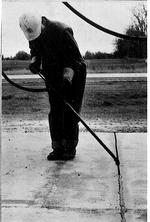
Figure 30 (bottom right). Sealing joint with hot-poured rubber-asphalt.
