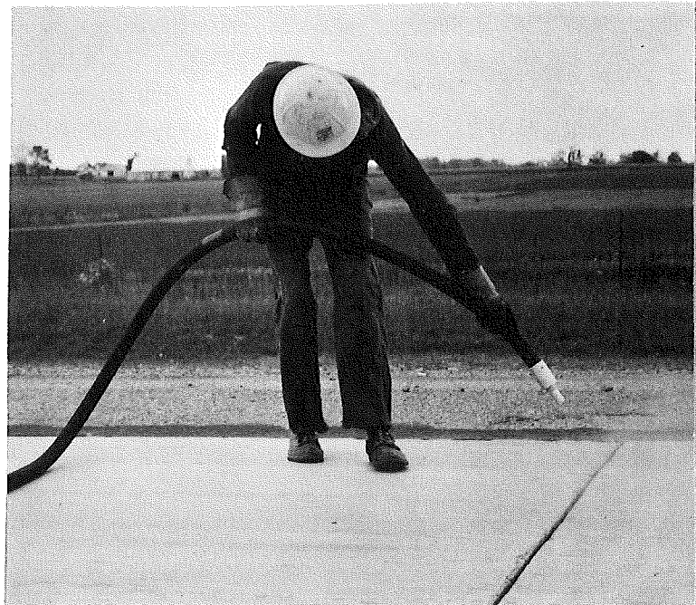
Figure 30 (bottom right). Sealing joint with hot-poured rubber-asphalt.
