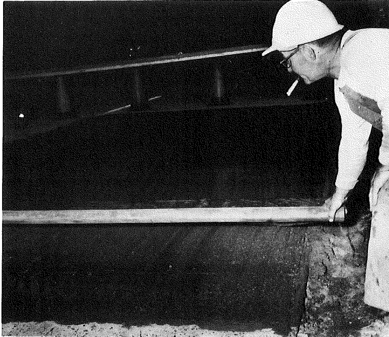
Figure 27 (top left). Applying burlap drag finish.
