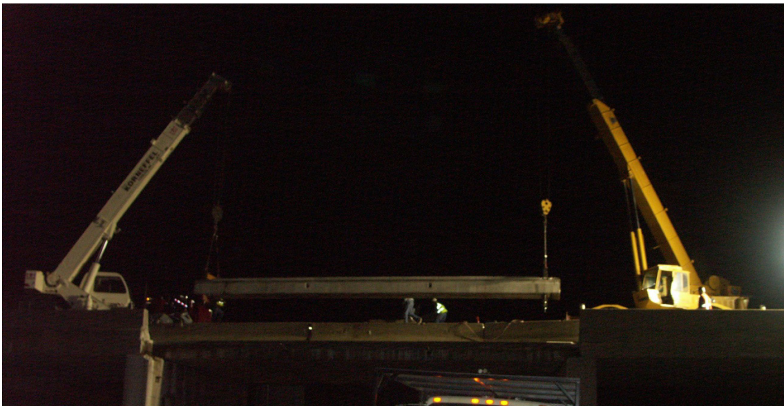
Photo 3-8. Lifting of the beam using two cranes
