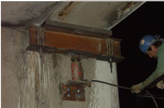
Photo 3-7. Force application using hydraulic jacks at both ends of the beam
