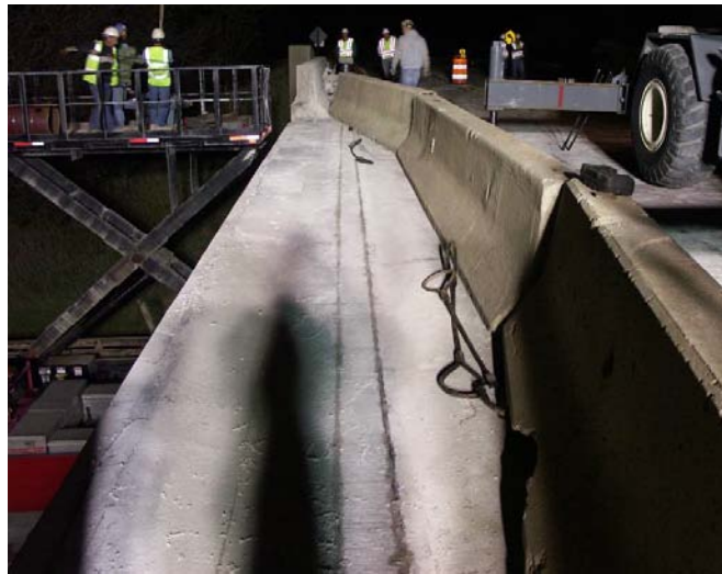
Photo 3-5. Saw cut at the exterior and interior beam joint
