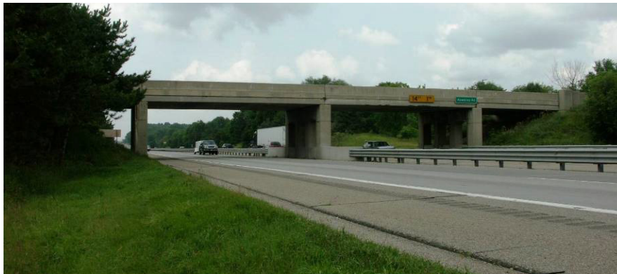
Photo 3-1. Bridge on Hawkins Road over I-94 (S11-38101)
