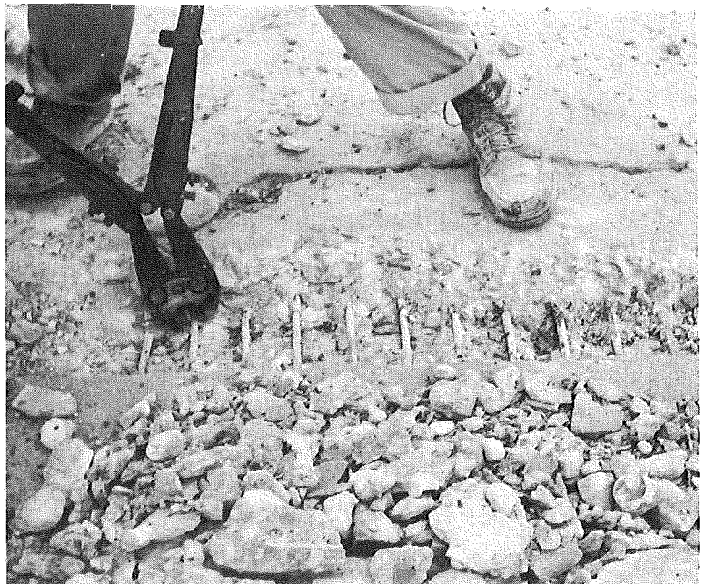
Figure 5. Cutting bar mat with acetylene torch (left), and welded wire mesh with wire cutters (right).
