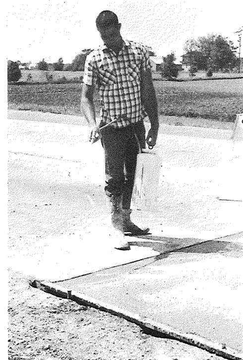
Figure 12. Application of white membrane curing compound (right).
