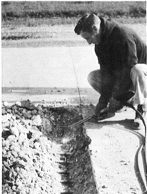
Figure 3. Breaking concrete with Arrow breaker.
