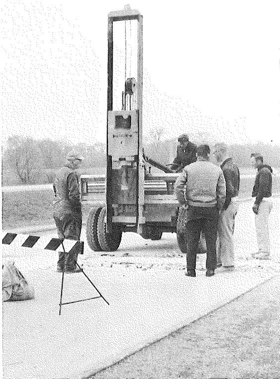
Figure 3. Breaking concrete with Arrow breaker.
