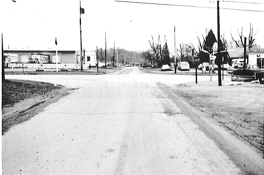
SOUTHBOUND WOODROW AVENUE
