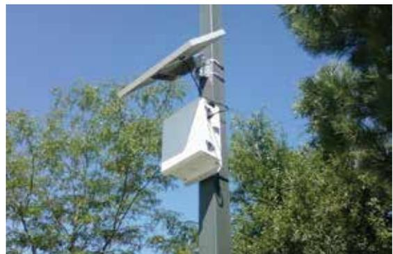
Figure 12: Photo. Example of a bluetooth antenna installation. (Source: JUB Engineers, Inc.)
