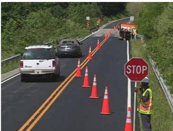
Figure 15: Manual flagging operations on low-volume two-lane roadways can have negative mobility impacts. (Source: FHWA)
