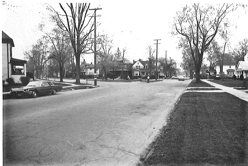
SOUTHBOUND NORTH AVENUE AT MARKET STREET
