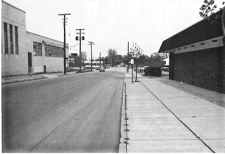
NORTHBOUND WALNUT STREET AT CLINTON STREET
