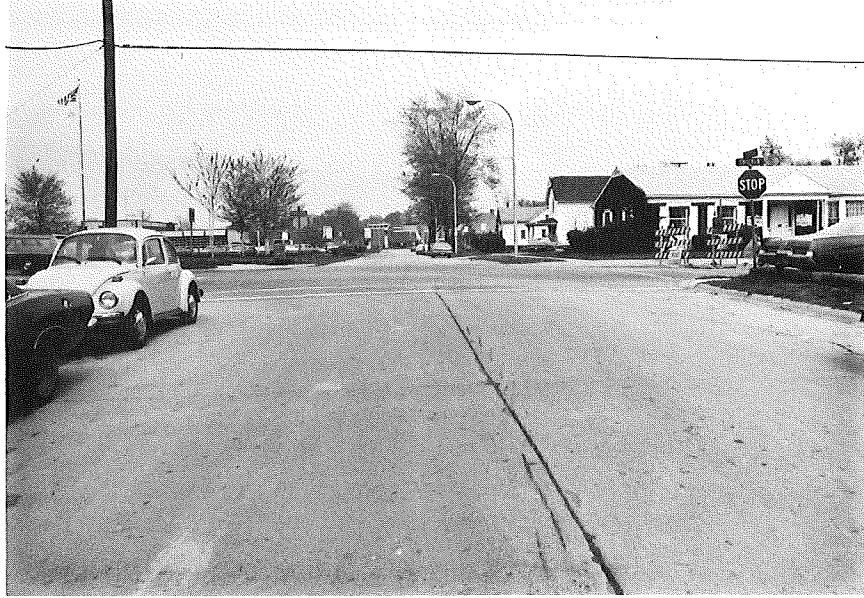
NORTHEASTBOUND FIRST STREET
