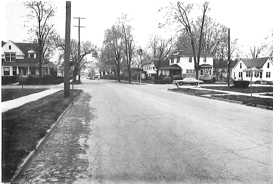
SOUTHBOUND NORTH AVENUE AT HUBBARD AVENUE
