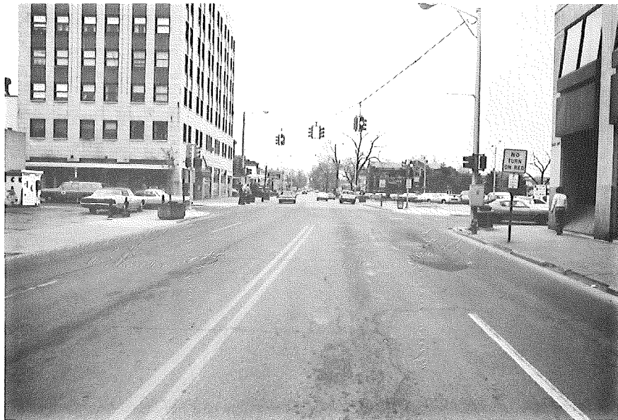
WESTBOUND CASS AVENUE
