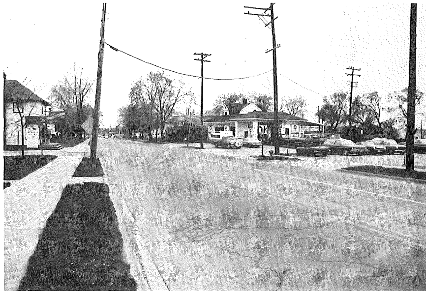
WESTBOUND CASS AVENUE
