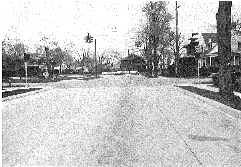
EASTBOUND HUBBARD AVENUE AT NORTH AVENUE
