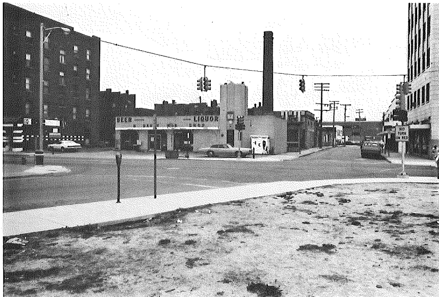
SOUTHBOUND WALNUT STREET
