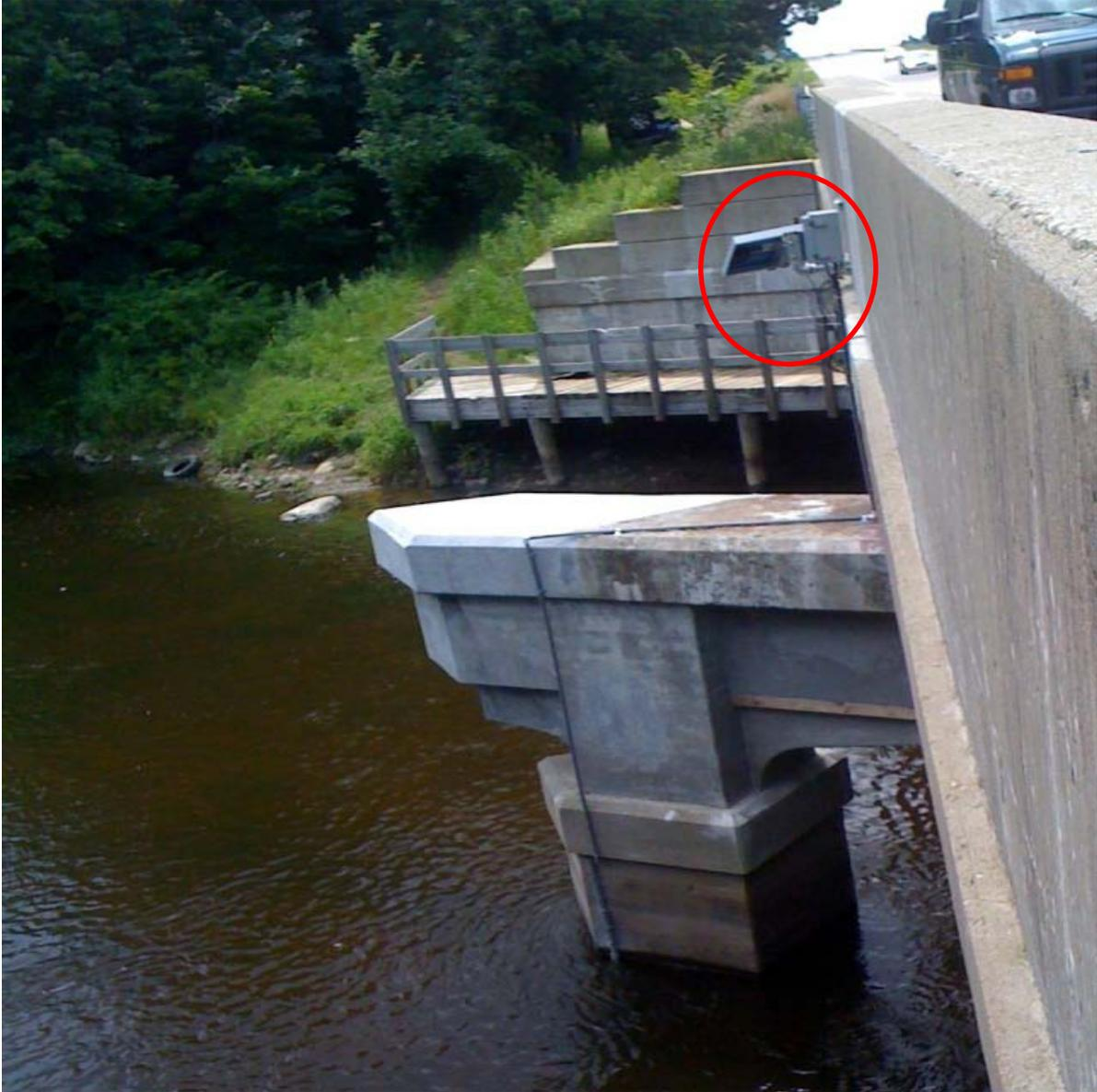
**Figure 8.26** Extended pier with data collection platform on the upstream side of bridge on M-99 over the Grand River
