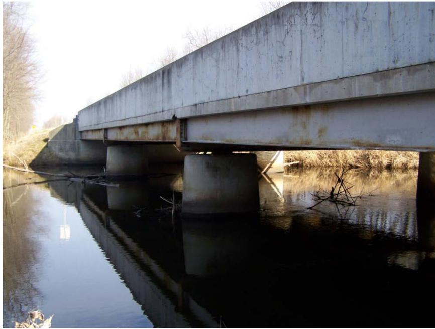
**Figure 8.20** Pine River at Lumberjack Road (south) with debris pile on north pier.
