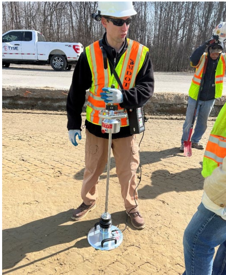
Figure 6.8. Light Weight Deflectometer Test on I-275.
