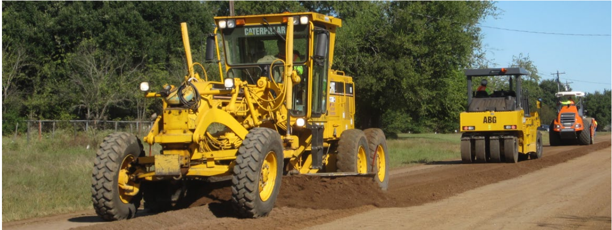
Figure 19. Finishing with a Blade Followed by Pneumatic and Smooth-Drum Steel Wheel Rollers
