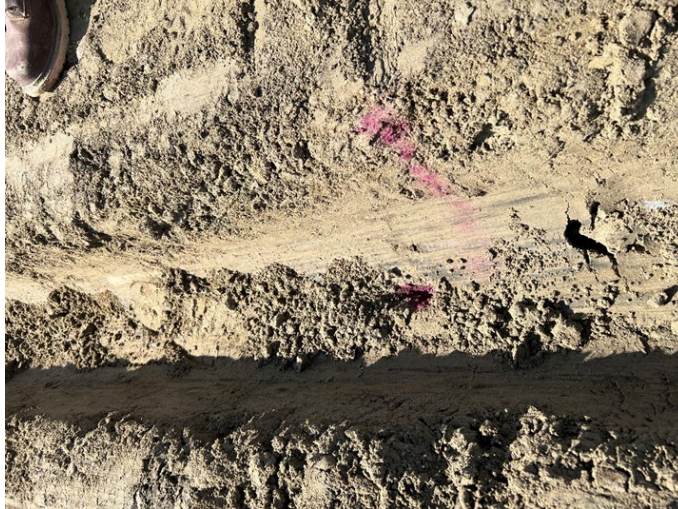
Figure 6.9. Depth Check Using Phenolphthalein Solution on I-275.
