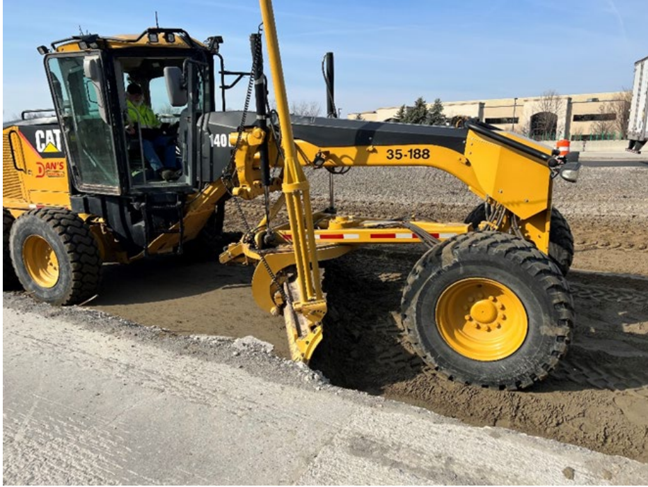
Figure 6.5. Grading with the Motor Grader on I-275.
