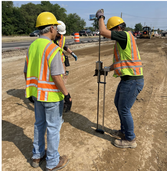
Figure 6.15. Dynamic Cone Penetration Testing on US-24.
