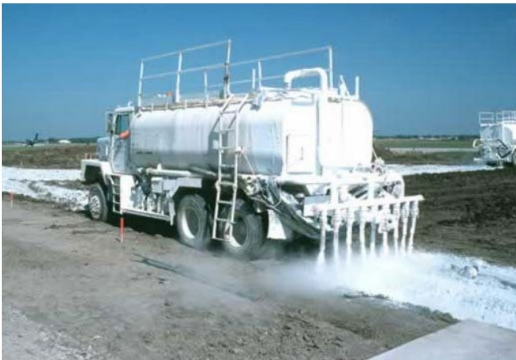
Figure 4. Lime Slurry Spreader or Distributor (NLA, 2004)
