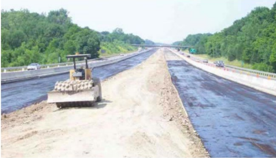
Figure 20. Prime Coat Emulsion for Curing (NLA, 2004)
