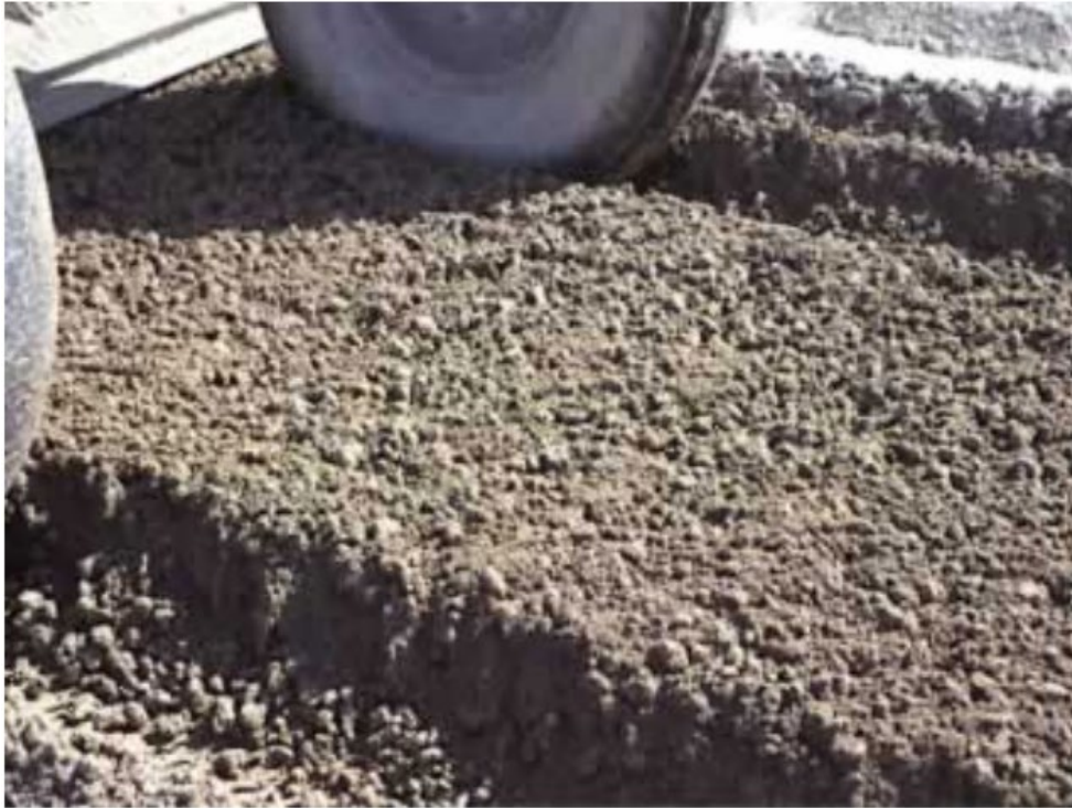
Figure 1. Lime-Treated Soils in Friable and Granular Condition (National Lime Association [NLA], 2004)
