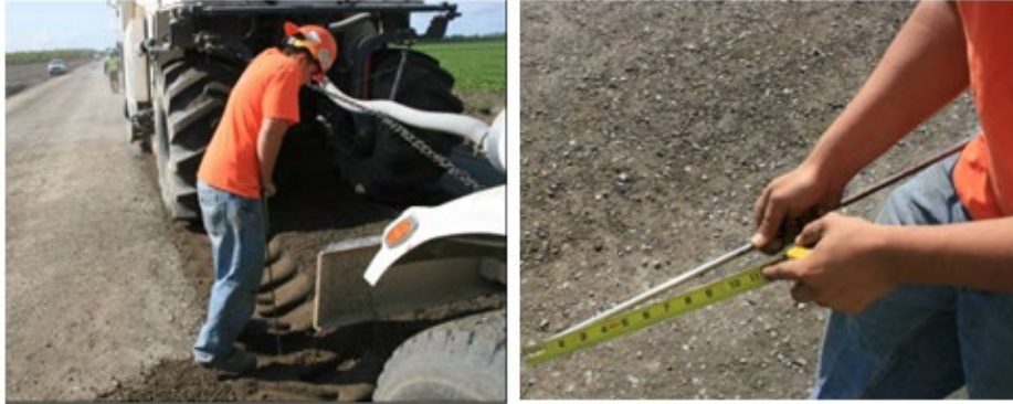
Figure 15. Checking Mixing Depth during Initial Mixing (Jones et al., 2010)
