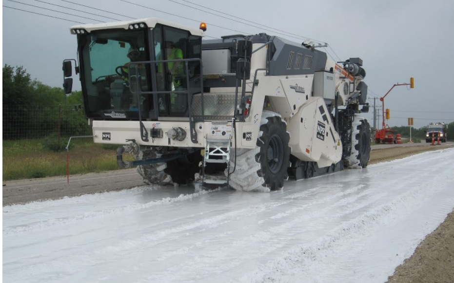
Figure 5. Rotary Pulvimixer Mixing in Lime Slurry
