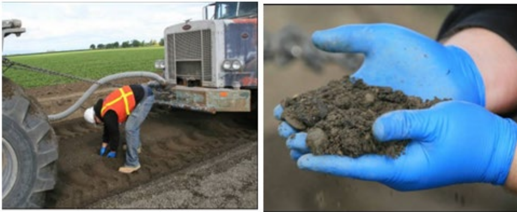
Figure 16. Visually Checking the Consistency of Mixed Materials (Jones et al., 2010)
