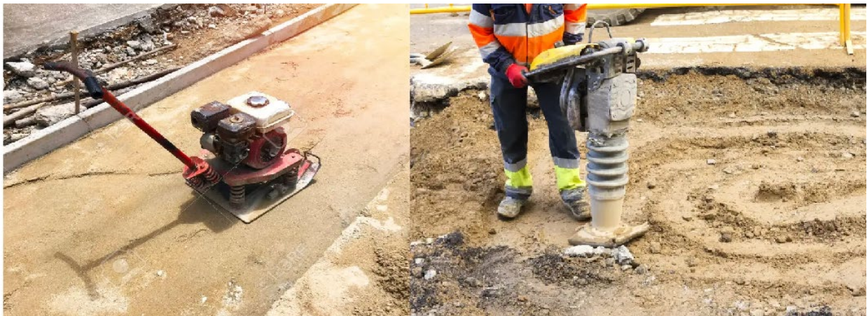
Figure 9. Plate Vibrator and Rammer/Tamper
