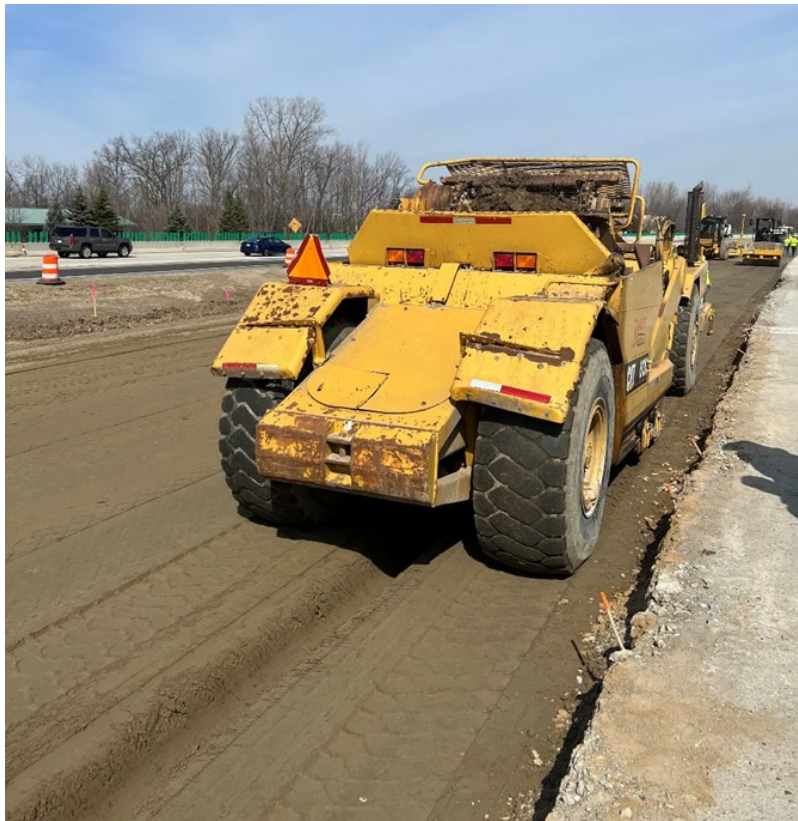
Figure 6.6. Underdrain Construction on I-275.
