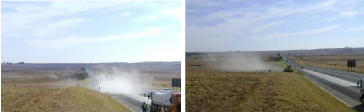
Figure 14. Dusting and Scattering of Cement due to Wind (Jones et al., 2010)
