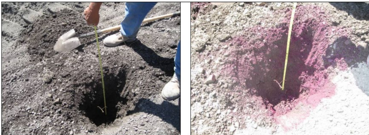
Figure 17. Checking Stabilizer Mixing Consistency and Depth Using Phenolphthalein (Jones et al., 2010)
