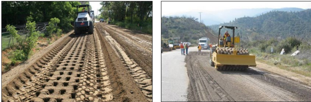
Figure 18. Use of Padfoot Rollers for Initial Compaction (Jones et al., 2010)
