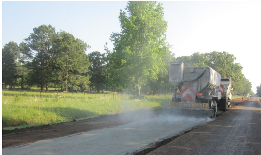
Figure 3. Quicklime/Cement Spreader or Distributor Spreading Portland Cement
