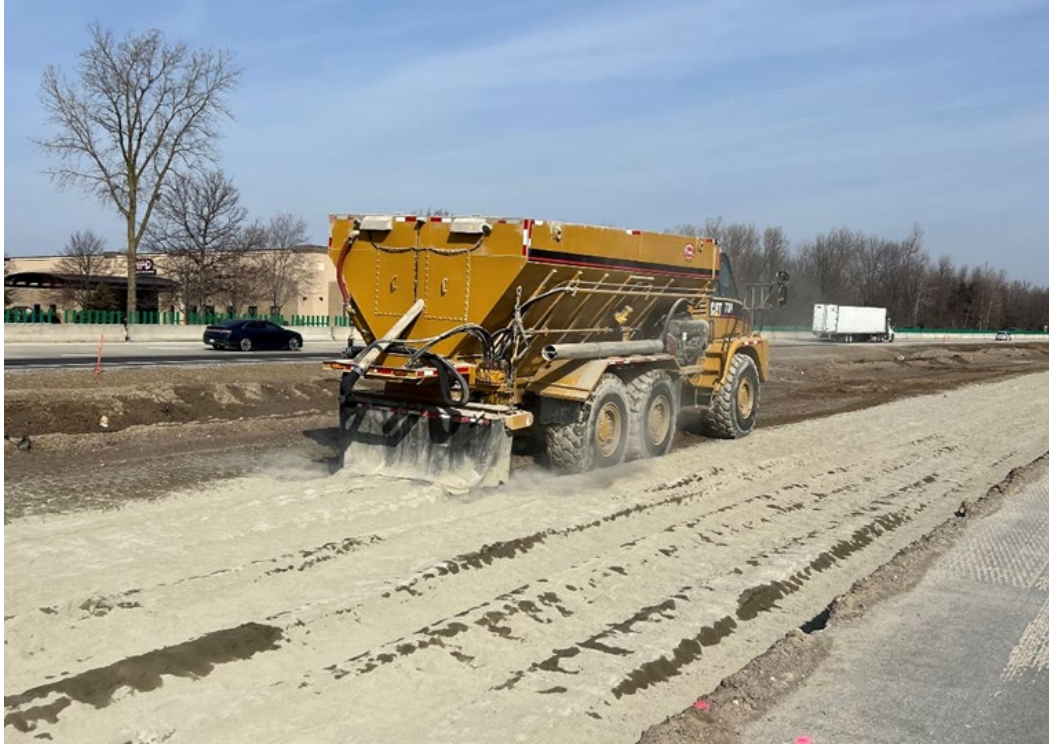
Figure 6.1. Spreading of Cement on I-275.
