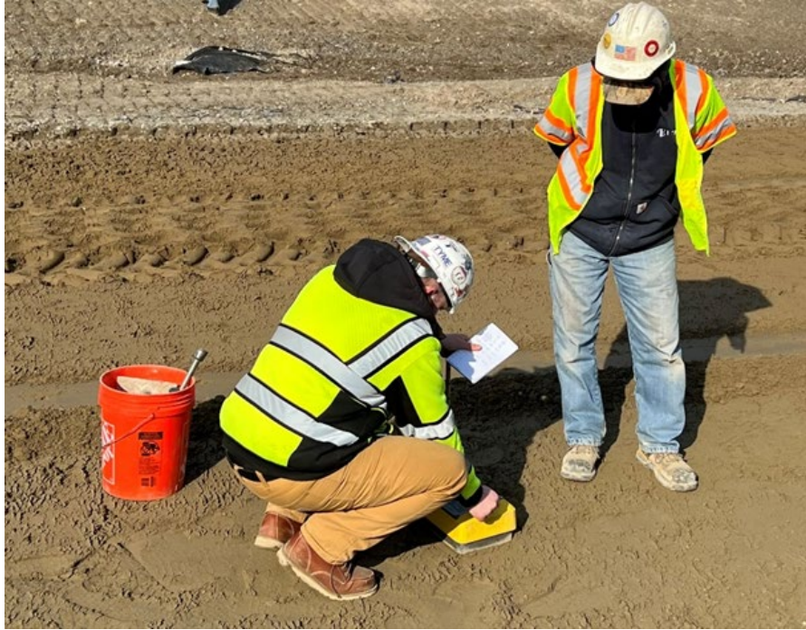
Figure 6.7. Nuclear Density Test on I-275.
