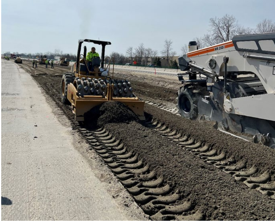
Figure 6.3. Rolling with Sheep Foot Roller on I-275.
