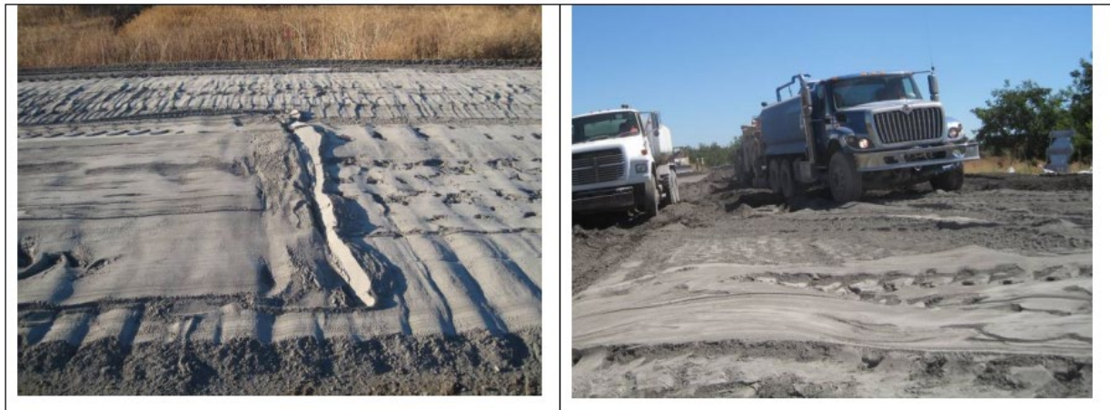
Figure 13. Uneven Distribution of Chemical Substances (Jones et al., 2010)
