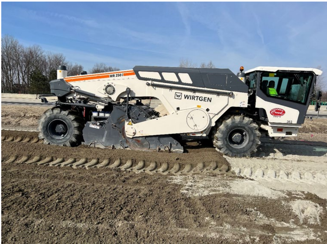
Figure 6.2. Pulverizing on I-275.
