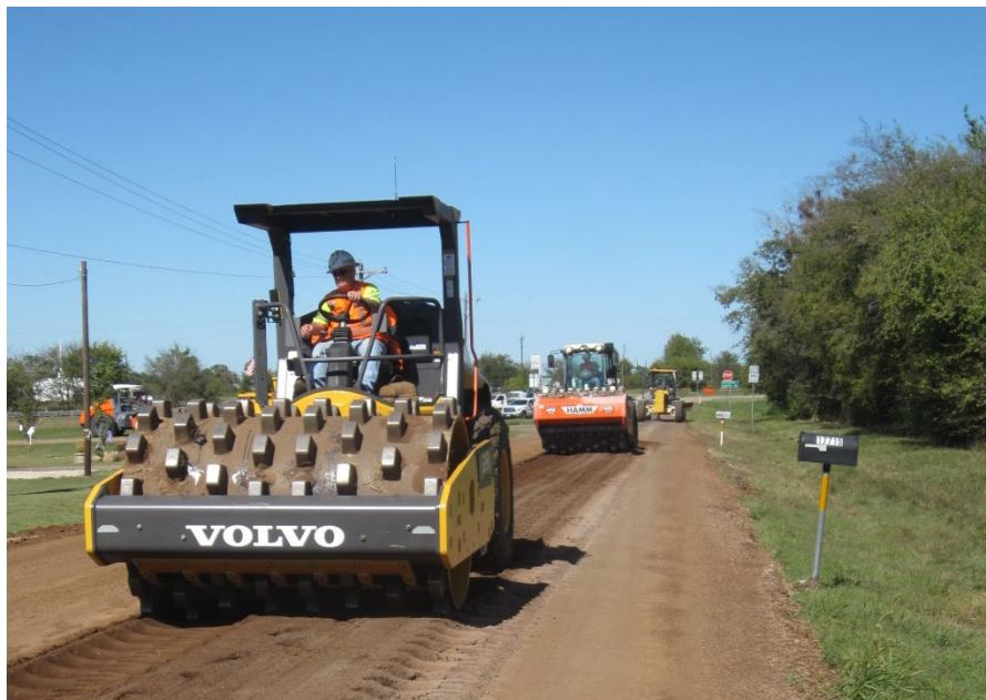
Figure 6. Sheepsfoot or Vibratory Padfoot Rollers
