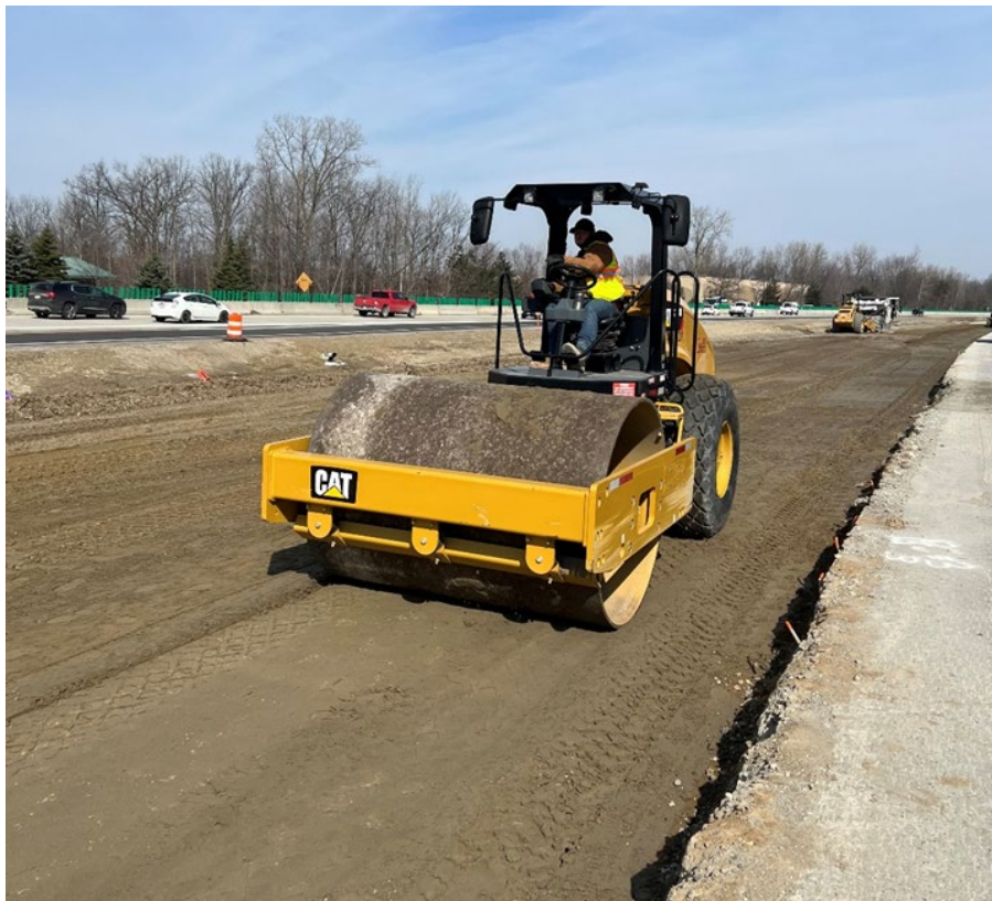
Figure 6.4. Rolling with Smooth Drum Rollers on I-275.
