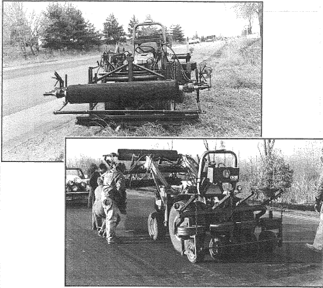
Figure 3. Modified tractor for installing the Glasgrid.
