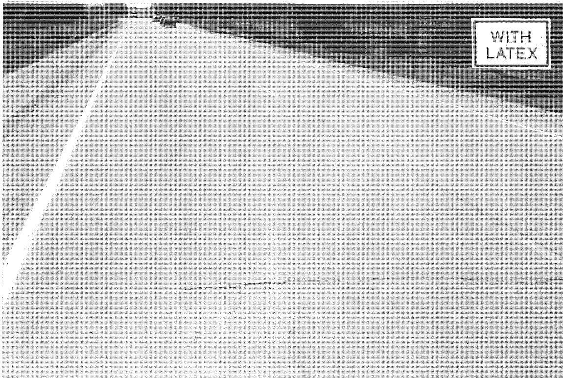
Figure 10 Typical condition of test area with bituminous separation course after 41 months of service.
