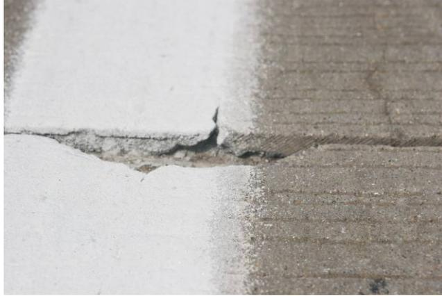
Figure 3.4 Longitudinal cracks at transverse joints initiate joint associated distress just below the tined surface.
