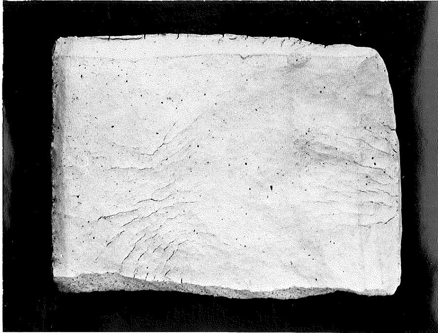
▲ Figure 2. Surface cracking in Perma-Line exposed outdoors for 3-1/2 months.
