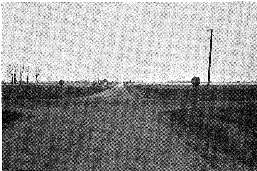
WESTBOUND ELMWOOD ROAD
