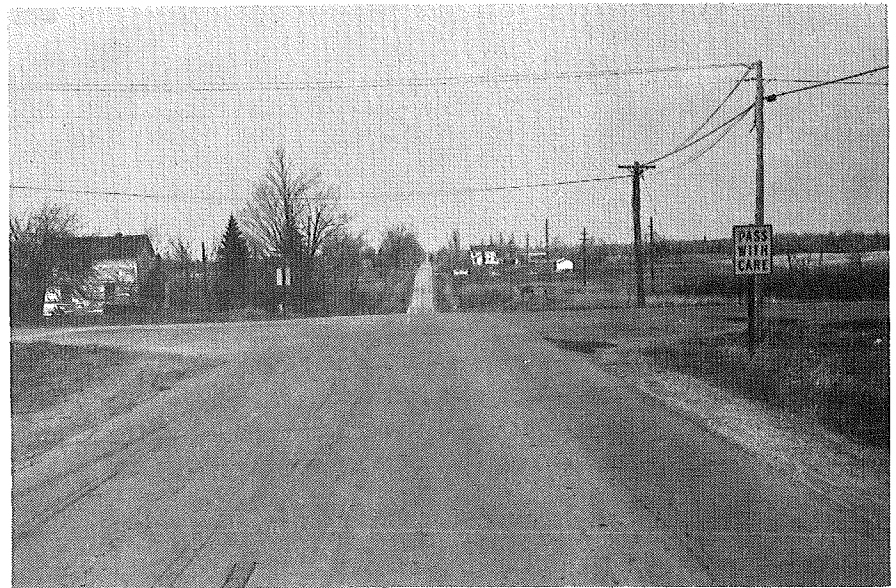
NORTHBOUND FOSTORIA ROAD
